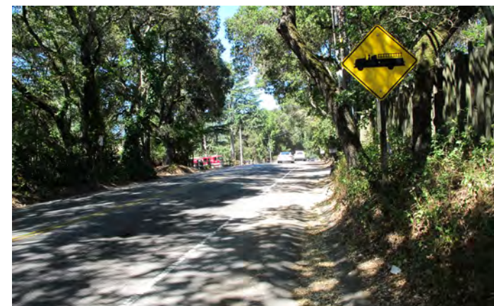
Looking west on Woodside Road, east of school: trees, utility poles and ground slope constrain widening for walkway.
