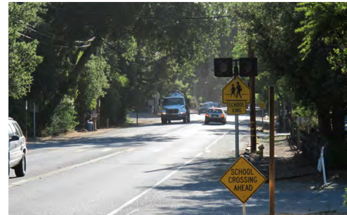
Looking east towards western crosswalk on Woodside Road; obsolete school area signing.
