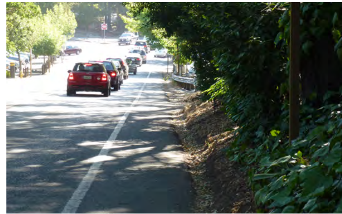
South side of Woodside Road approaching Town Center: lack of separated walkway.
