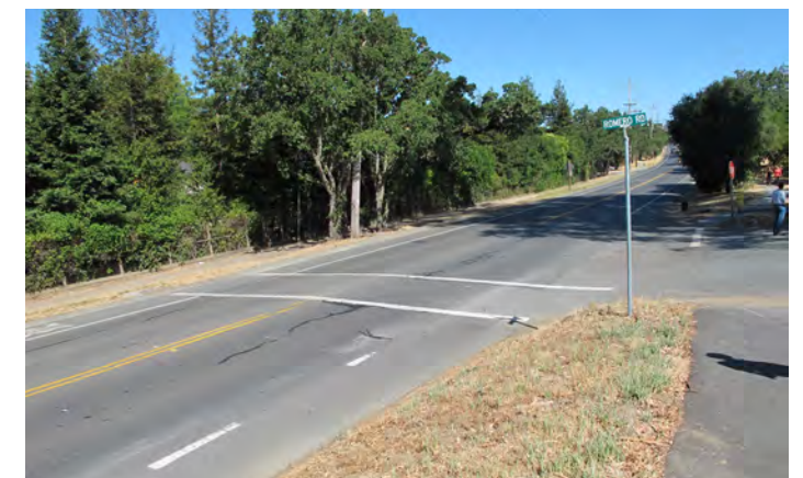
Crosswalk across Cañada Road at Romero Road; standard crosswalk without signing, curb ramps, and connection to pathway on west side of roadway.
