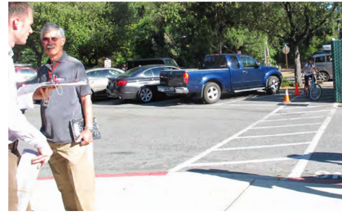
Crosswalk across school parking lot; sight issues and lack of curb ramps.
