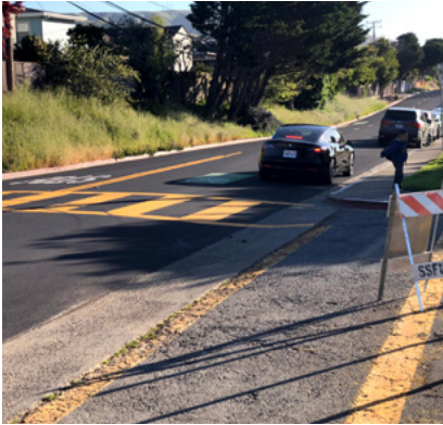
Figure 7. Missing sidewalk on the north side of Ponderosa Rd east of Lassen St.
