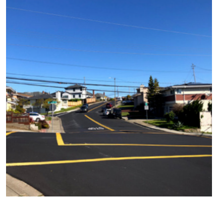
Figure 6. Wide turning radii at the Alida Way/Fairway Dr and Ponderosa Rd intersection (looking north towards Fairway Dr).
