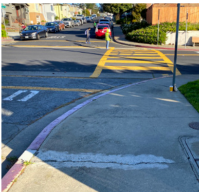
Figure 1. No curb ramps on the southeast corner at Lassen St and Ponderosa Rd (looking north across Ponderosa Rd).
