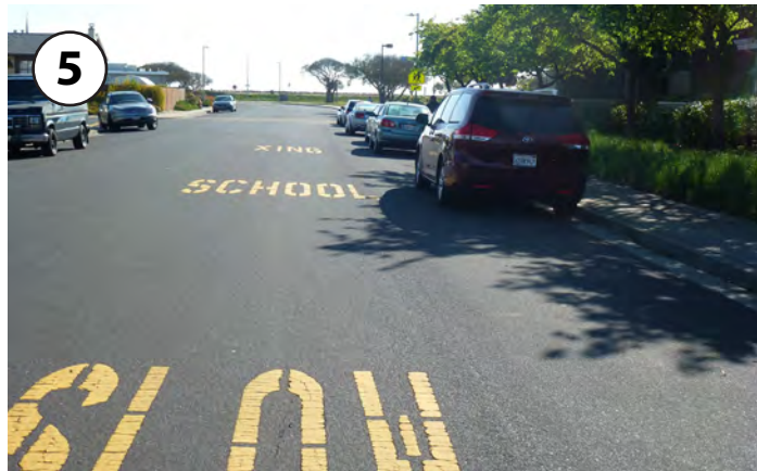
5 SLOW SCHOOL XING pavement stencils signal that an uncontrolled crosswalk is ahead.
