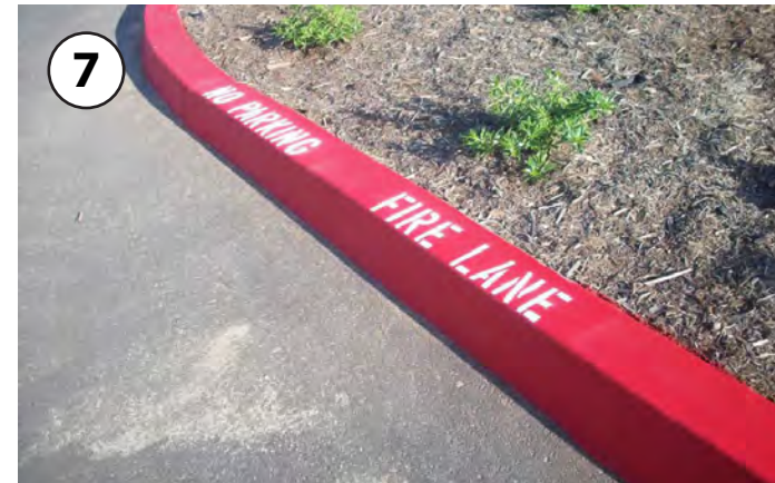
7 Red curb paint delineates areas where parking is prohibited.
