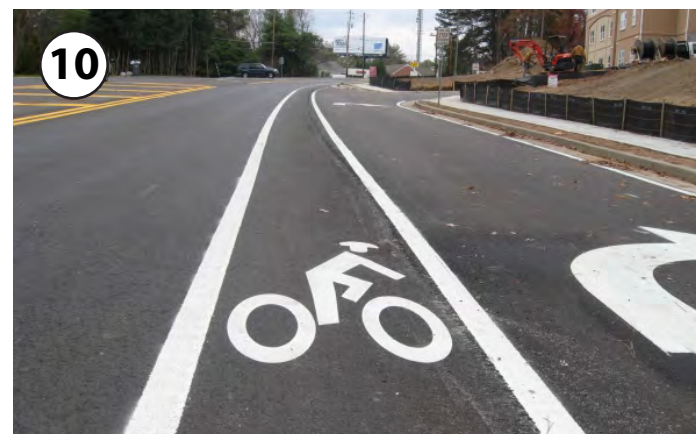
10 Restriping traffic, bicycle, and parking lanes that have faded can assist school traffic operations.
