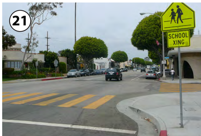
21 Increasing the size of the pedestrian waiting area can keep sidewalks accessible.
