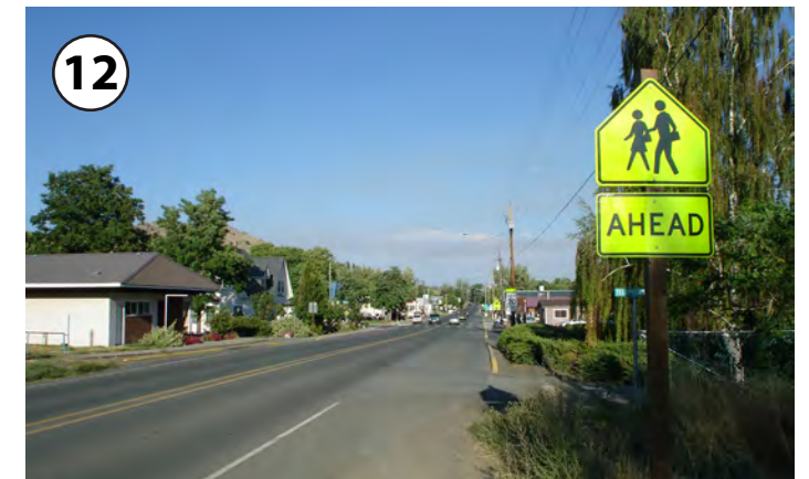
12 Assembly B and D signage alert motorists to an uncontrolled crosswalk ahead.
