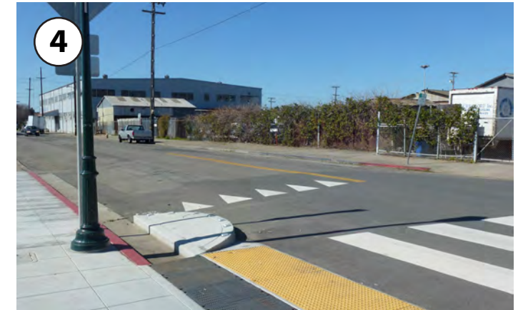
4 Advance yield lines/sharks teeth instruct motorists where to yield at uncontrolled crosswalks.
