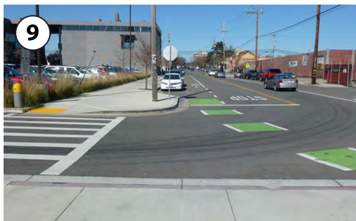
9 Enhanced bike lanes can be used for conflict zones, where motorist and bicycle paths cross.
