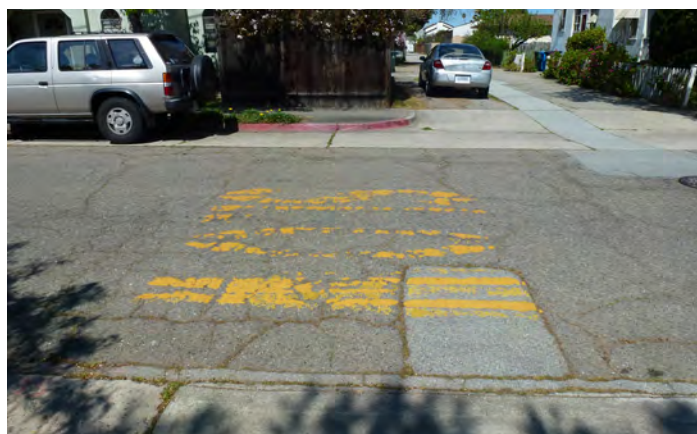
Signage and stenciling should be upgraded and restriped at many locations around the school site.
