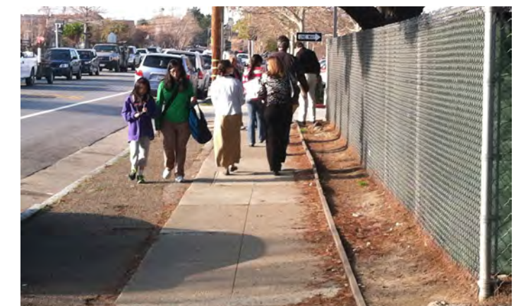
Sidewalk repair or widening could improve walking conditions.
