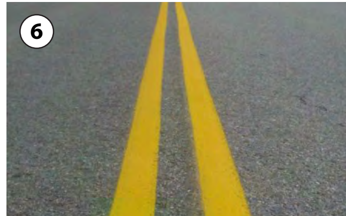
6 Double yellow centerlines discourage U-turns by motorists.
