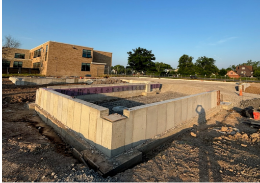
New UPK Addition @WBS - Foundations
