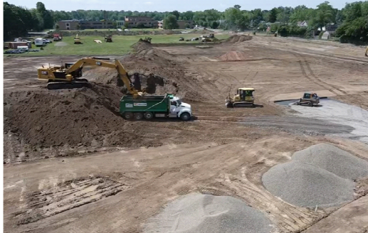
Turf Complex - Stripping Topsoil and Laying Down Stone
