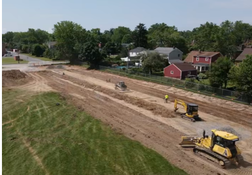
Turf Complex - Stripping Topsoil
