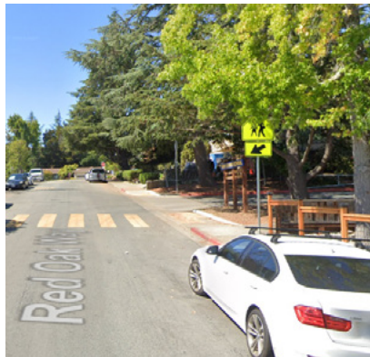
Figure 8. Obstructed pedestrian crossing sign at midblock crossing on Red Oak Way
