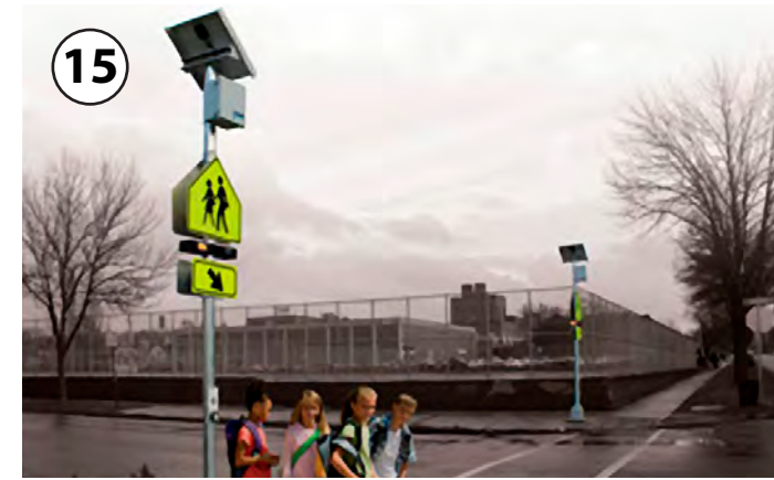
15 Rectangular Rapid Flash Beacons increase yield compliance at uncontrolled crossings.
