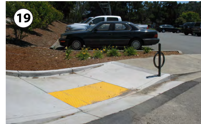
19 Curb ramps provide access to disabled pedestrians and parents walking with strollers.
