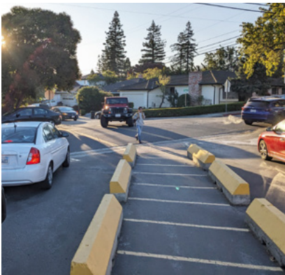
Figure 7. Crosswalk that ends in the driveway between two lanes of vehicles is a high conflict crossing.
