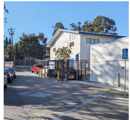
Figure 9. Parking lot to the south of the driveway does not have clear pedestrian space beyond the metal fencing shown.
