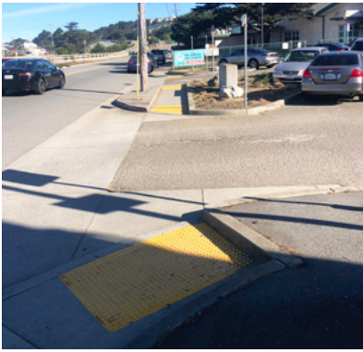
Figure 1. No crosswalks across the school parking lot driveways.
