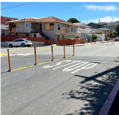
Figure 13. An example of a hardened centerline (see recommendation 3b).
