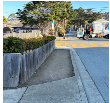
Figure 6. Missing sidewalk on Fremont Ave between Monterey Rd and Nelson Ave.
