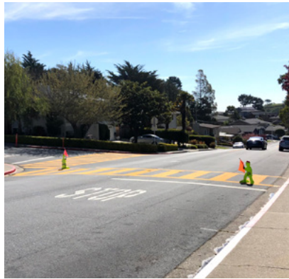
Figure 8. Missing curb ramps at Helen Dr/Banbury Ln
