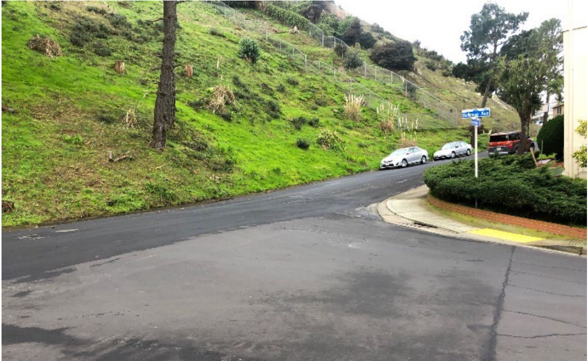
Existing conditions at the intersection of South Hill Boulevard and Ardendale Drive.
