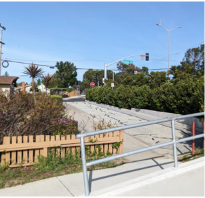
Figure 2. Dead end street between Tahoe Dr and school's driveway entrance
