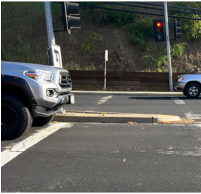
Figure 9. Noncompliant median in crosswalk presenting an opportunity for a pedestrian refuge island.
