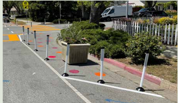
Quick Build Curb Extensions
