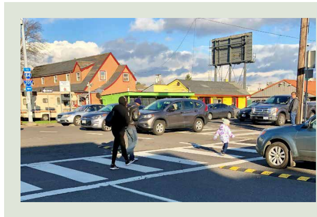
Hardened Centerlines Source: Portland Bureau of Transportation
