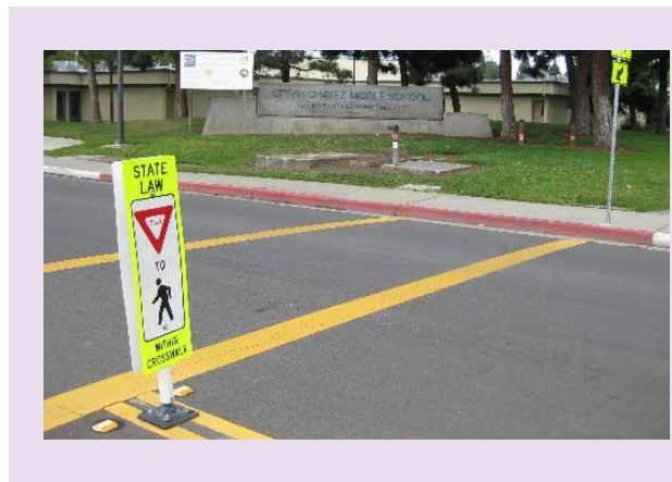
In-Street Pedestrian Crossing Signs
