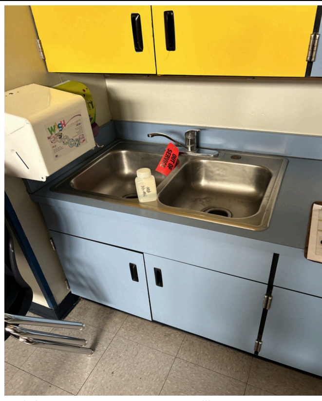
7/3/2024 - 1400-44 - Manor Hill - 001040-Room 31
