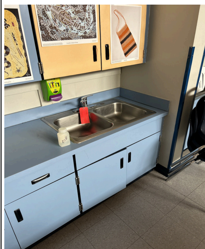
7/3/2024 - 1400-43 - Manor Hill - 00139-Room 31
