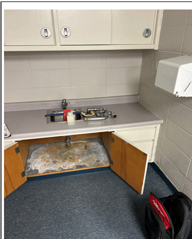
7/3/2024 - 1400-2 - Manor Hill - 001035-Room 9
