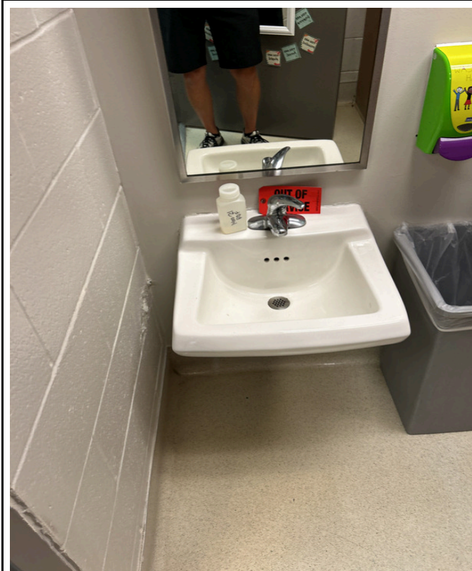
7/3/2024 - 1400-21 - Manor Hill - 001006-Room 14-Restroom
