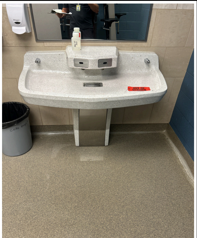
7/2/2024 - 1000-341 - Liberty North - 003950- Cafeteria-Boys Restroom
