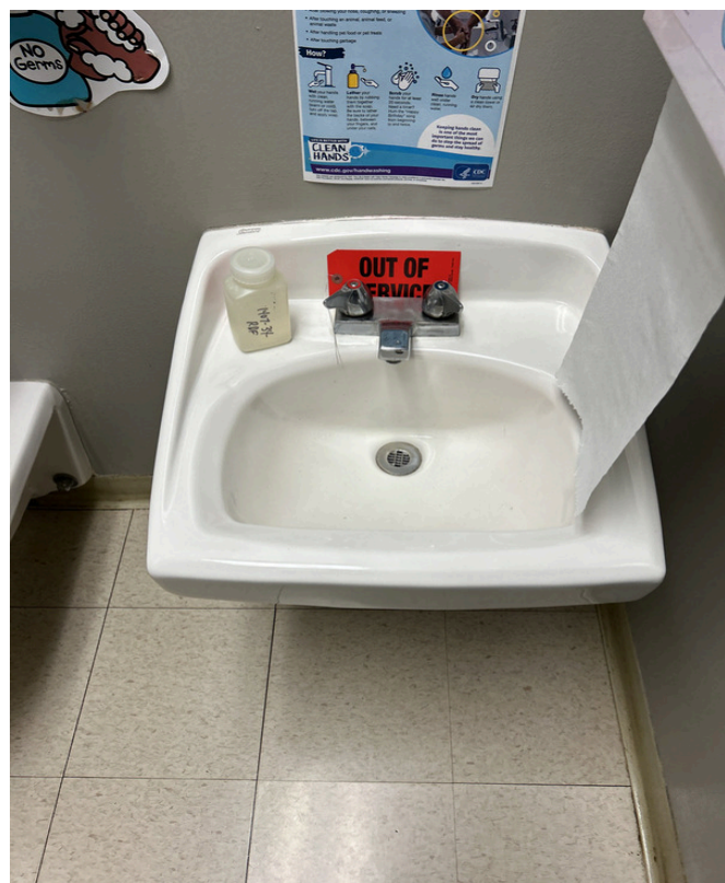
6/28/2024 - 1407-34 - Lewis and Clark - 001281- Room 44-Restroom-Left
