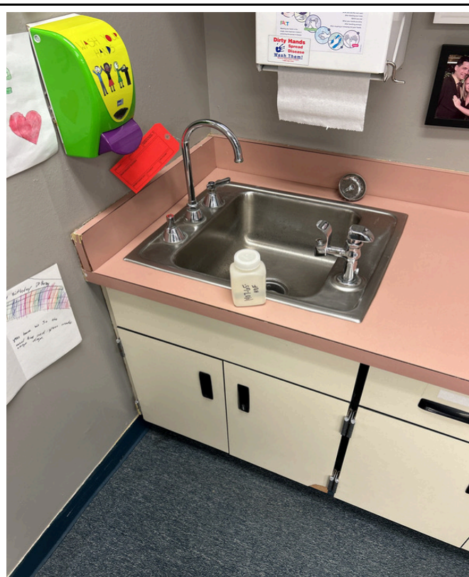
6/28/2024 - 1407-65 - Lewis and Clark - 001250F-Room 35
