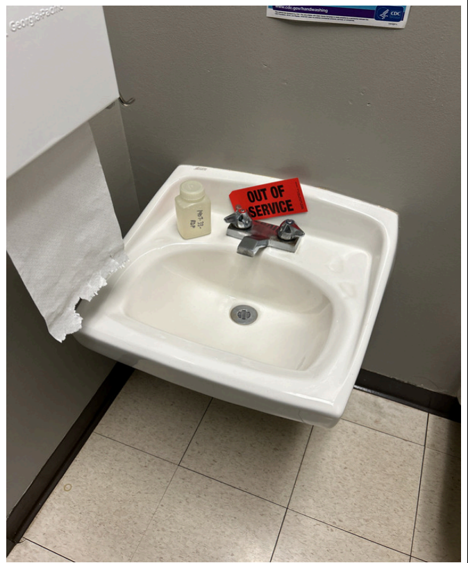
6/28/2024 - 1407-33 - Lewis and Clark - 001280- Room 44-Restroom-Right
