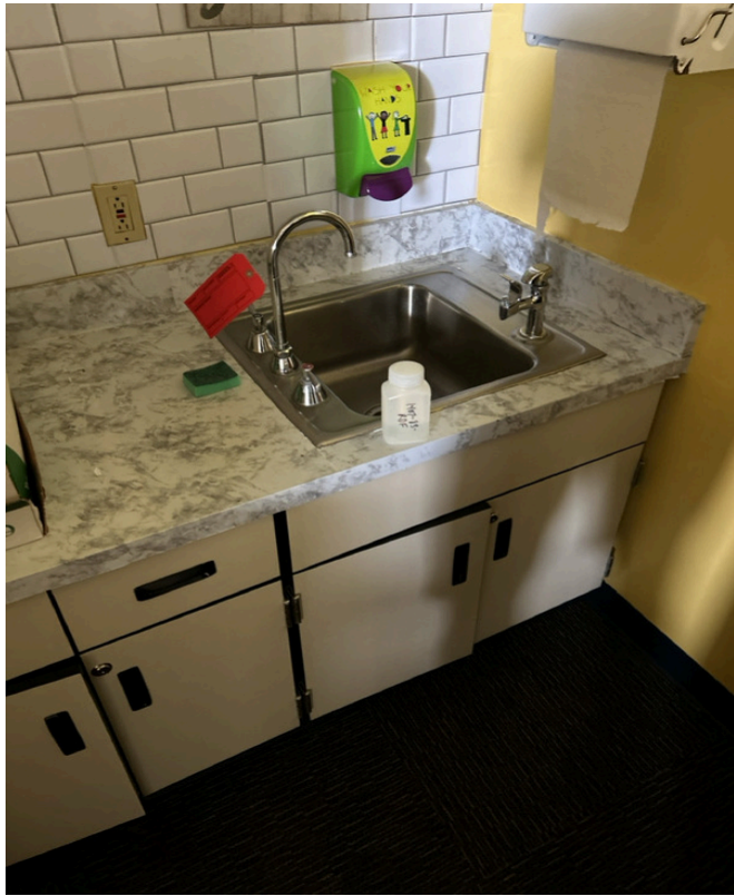
6/28/2024 - 1407-83 - Lewis and Clark - 001247F-Room 25
