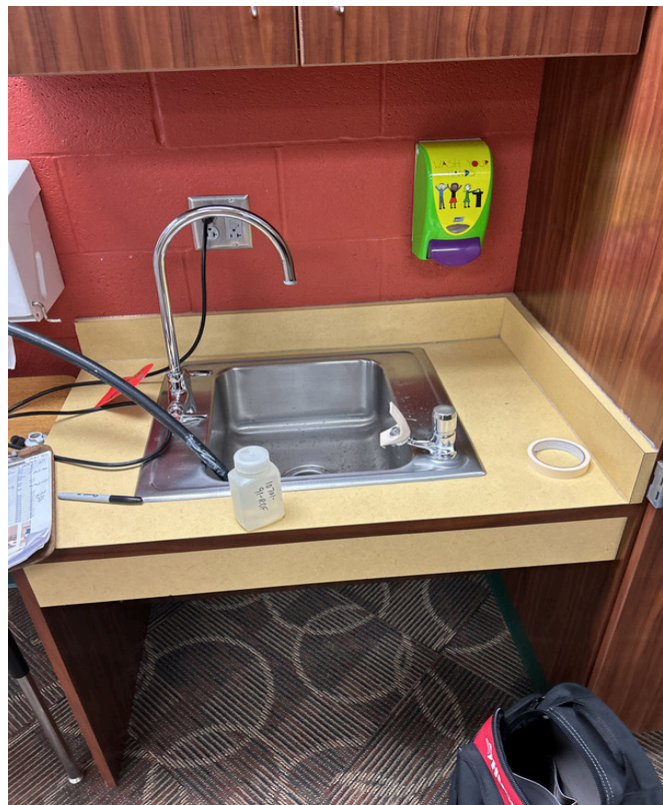
7/2/2024 - 10701-91 - Kellybrook Elementary - 001470F-Room 306
