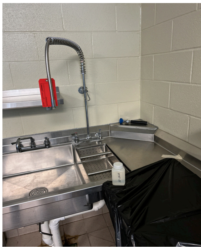
7/2/2024 - 10701-24 - Kellybrook Elementary - 004636-Kitchen-Outside Office-South
