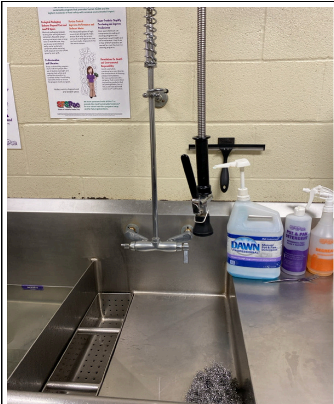
2/13/2025 - 10701-28 - Kellybrook Elementary - 004646-Kitchen-3 Bay Sink
