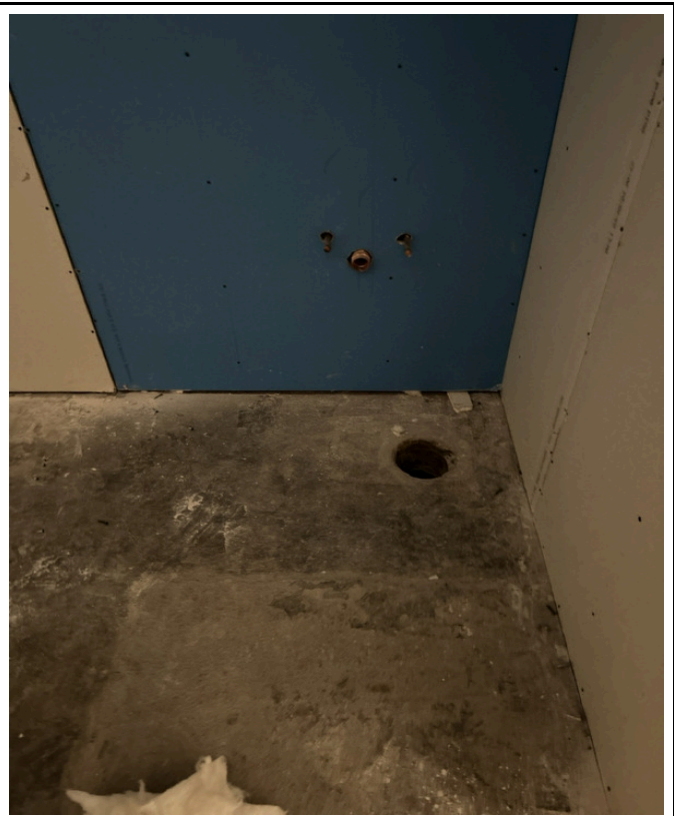
6/28/2024 - 201-22 - Franklin Elementary - 002568-Room 14 - Source Demolished
