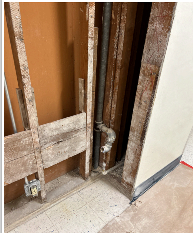
6/28/2024 - 201-34 - Franklin Elementary - 002567-Hall by Room 26 - Source Demolished
