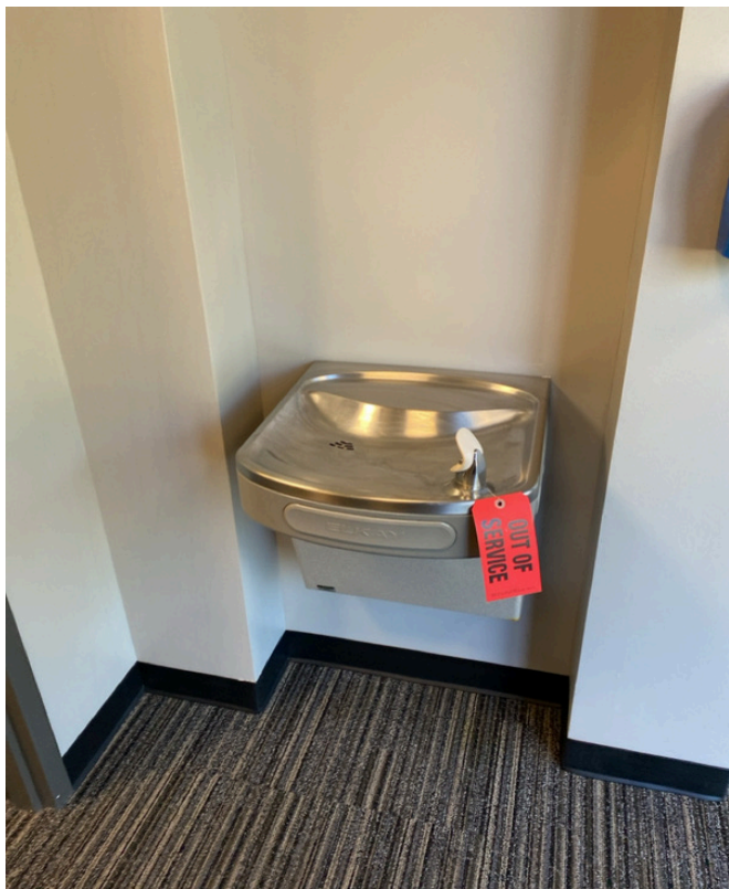
9/4/2024 - 8-33 - District Administration Center - 004544B-By Elevator 1st Floor
