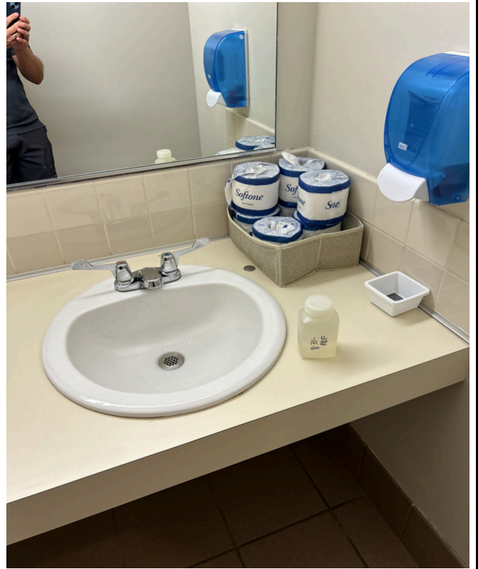
6/28/2024 - 8-31 - District Administration Center - 004547-By Elevator 1st Floor-Girls- Right
