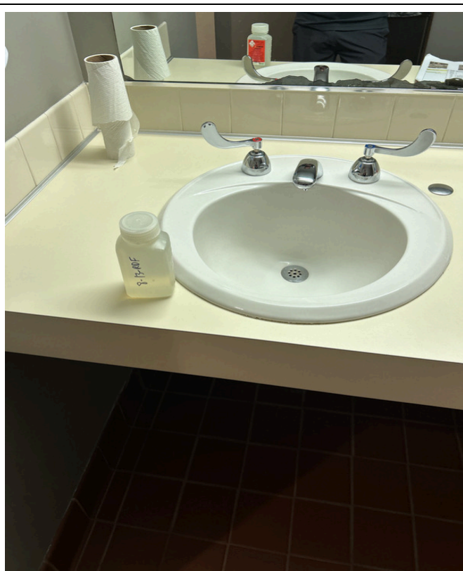
6/28/2024 - 8-13 - District Administration Center - 004560-By Elevator 3rd Floor-Boys-Left
