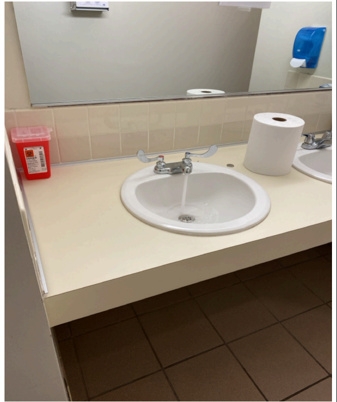
9/4/2024 - 8-32 - District Administration Center - 004548-By Elevator-1st Floor-Girls Left
