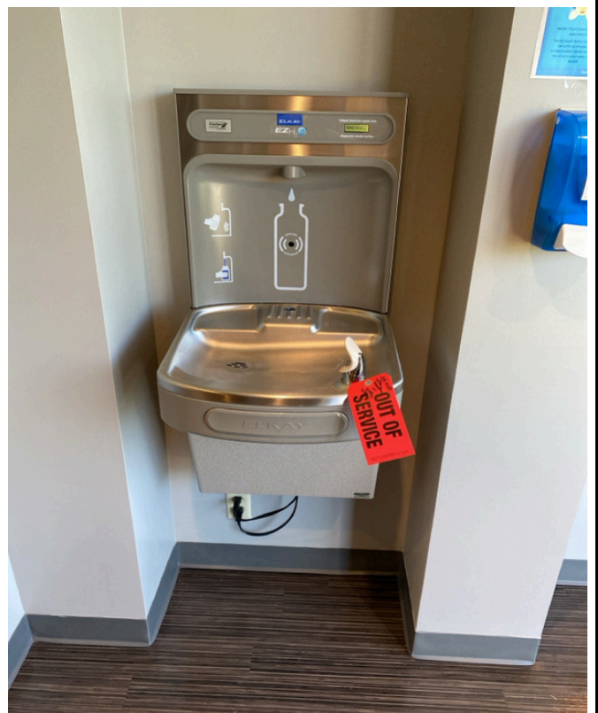
9/4/2024 - 8-1 - District Administration Center - 004563B-By Elevator 4th Floor
