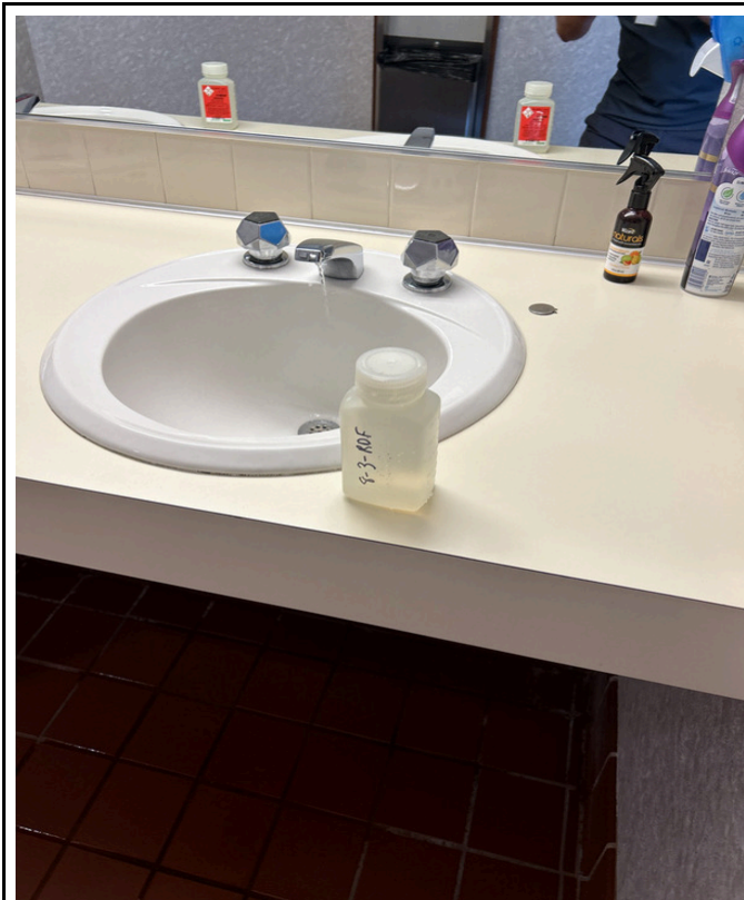
6/28/2024 - 8-3 - District Administration Center - 004564-By Elevator 4th Floor- Boys-Right
