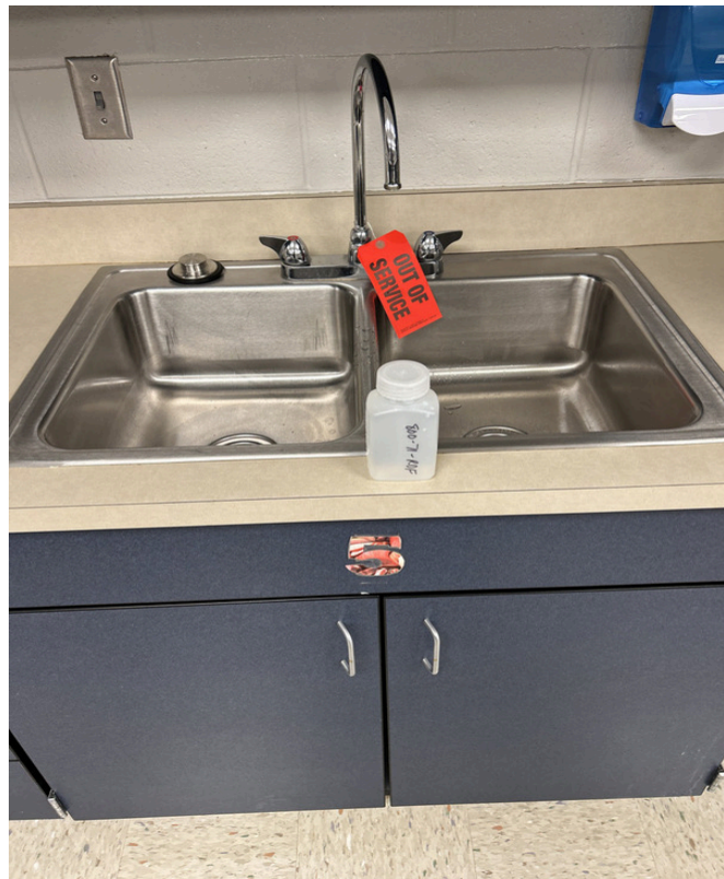
6/27/2024 - 800-71 - Discovery Middle School- Classroom 206 - 004257-Room 206-Kitchen 5
