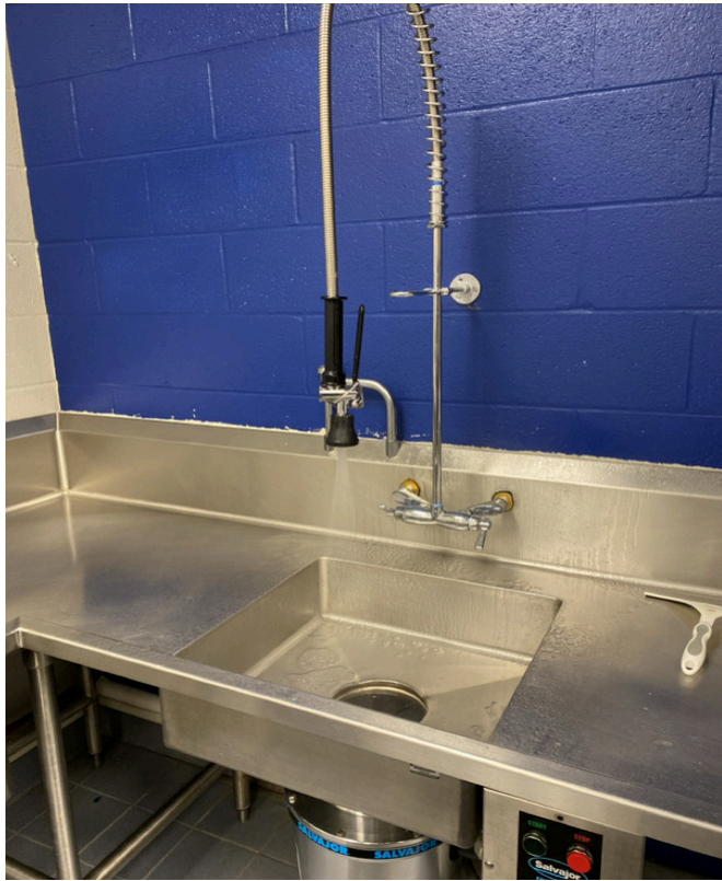
3/14/2025 - 800-148 - Discovery Middle School -004696-Kitchen-South Wall
