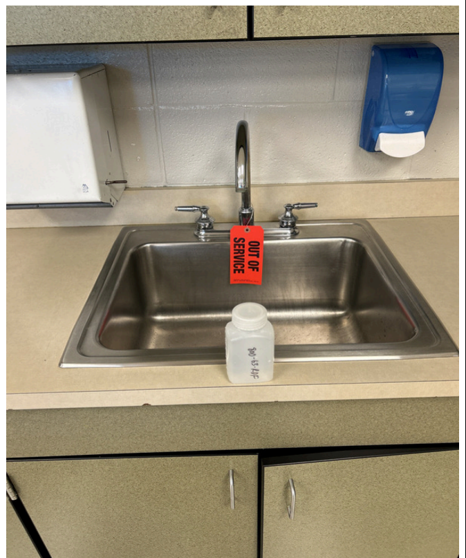
6/27/2024 - 800-63 - Discovery Middle School- Classroom 207 - 004261-Room 207-South Wall- Right Sink
