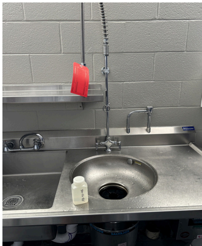
6/27/2024 - 800-146 - Discovery Middle School- Kitchen - 004694-Kitchen-East Wall
