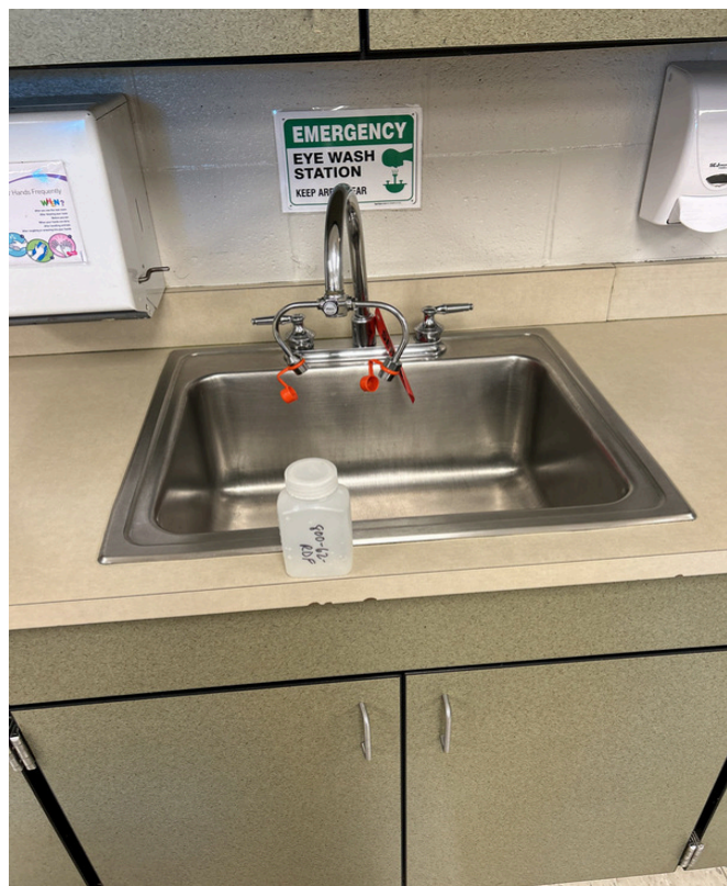
6/27/2024 - 800-62 - Discovery Middle School- Classroom 207 - 003202-Room 207-South Wall- Left Sink
