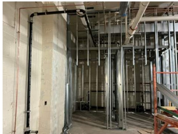
Framing at new bathrooms and MEP
