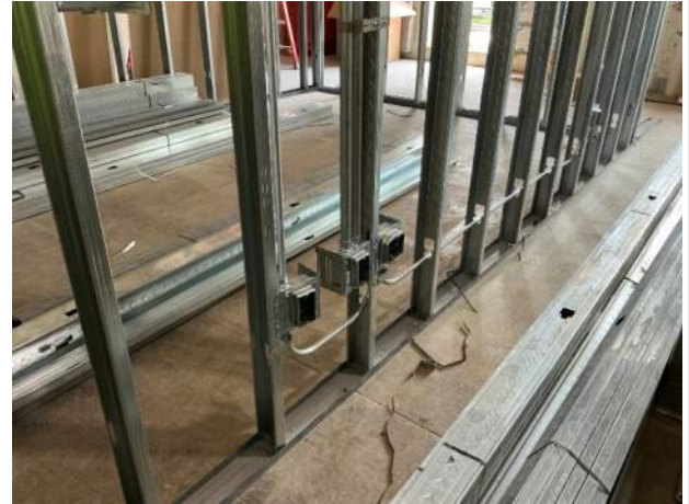
Lab electrical rough-ins
