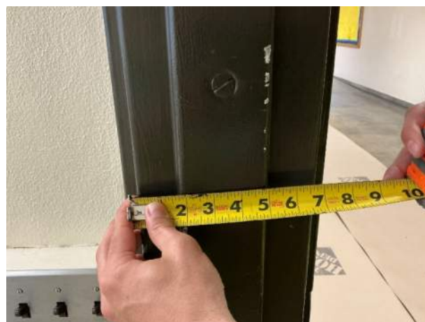
Reviewed existing door frame depths and trim to coordinate for new frames in existing walls
