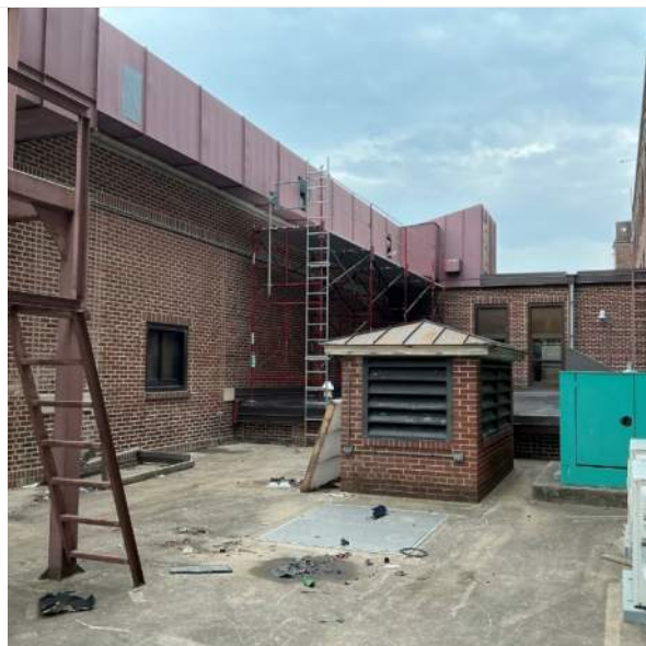
Exterior scaffold for dust collector demolition
