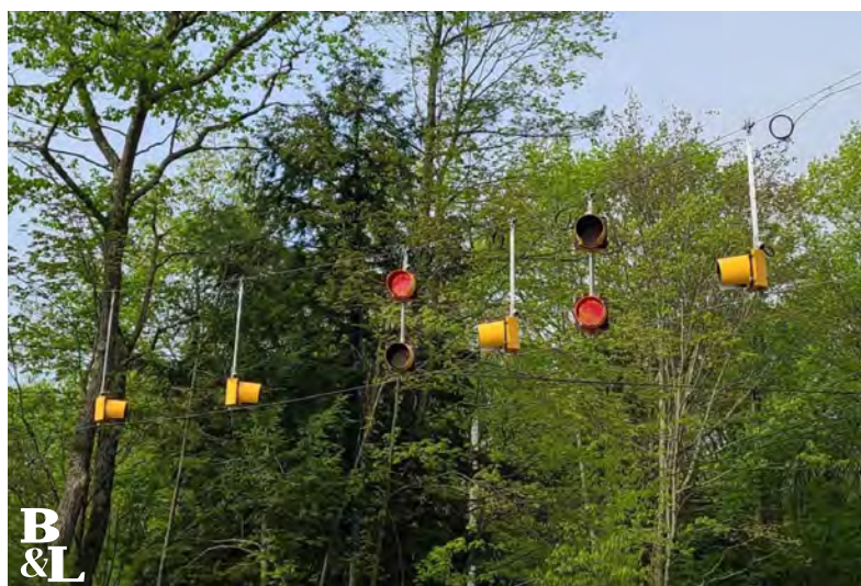
Figure 25 - Example of a Newer Flashing Beacon Design
