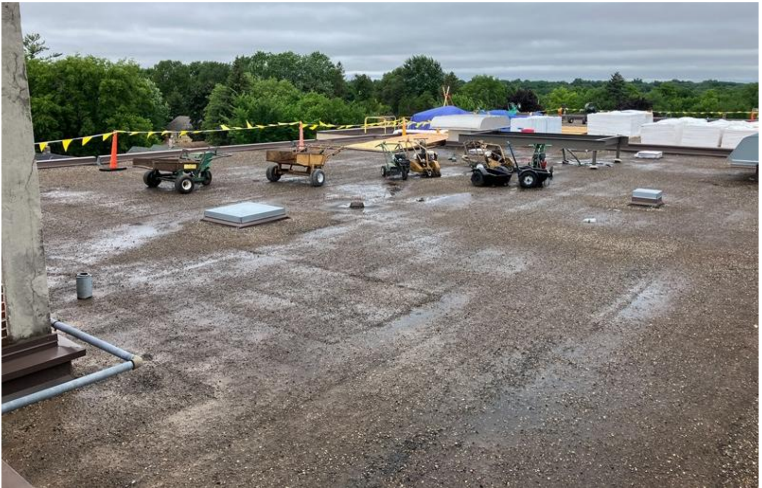
From top left: Prepping for new radiators; exposed shaft; open ceiling for HVAC; one roof underway (June 2025)
