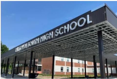
RSHS: Construction continues for new canopy
