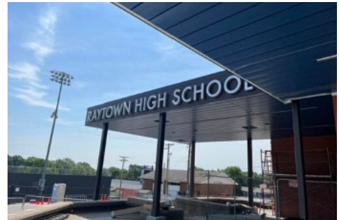
RHS: Work-in-progress during signage update
