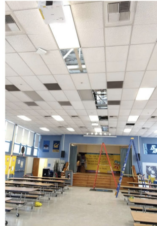
Conduit Installation above Rosa Parks Cafeteria Ceiling
