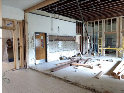
Photo during construction 3
