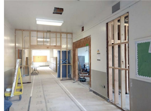
Reconstruction of Entrance Lobby (During Construction)
