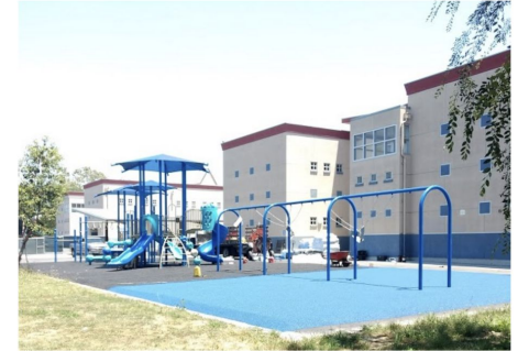
Primary Playground Equipment in final stages of construction
