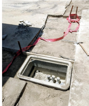
Fire Alarm Conduit boxes prior to backfill with asphalt paving
