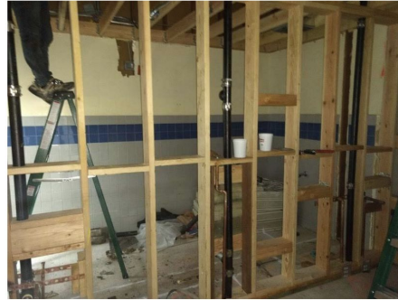
Staff Restrooms During Construction
