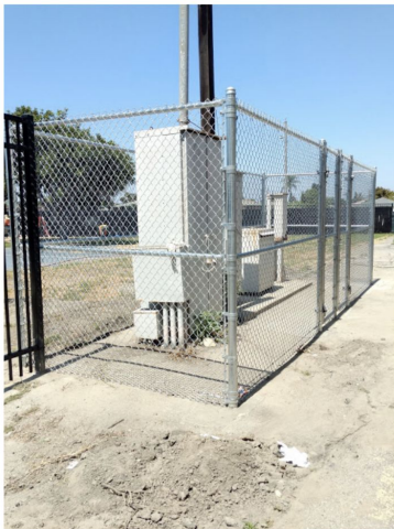
Replaced Electrical Equipment Enclosure
