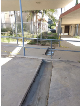
Slurry Backfill of Trenches at Abbott ES after conduit installation
