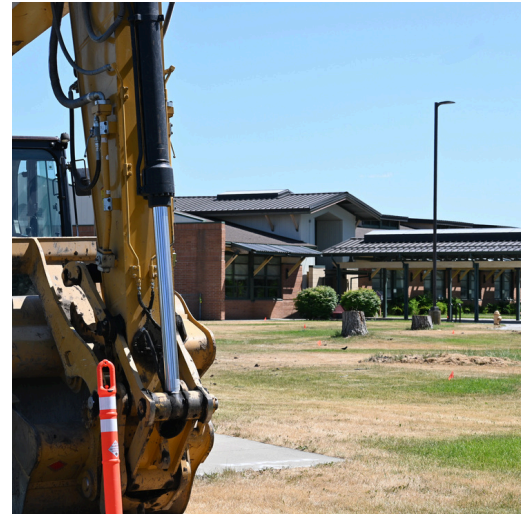
The construction area is flagged and prepped at Windsor Elementary for the new bus loop.
