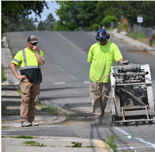
Construction crews prep the worksite at Salnave Elementary.
