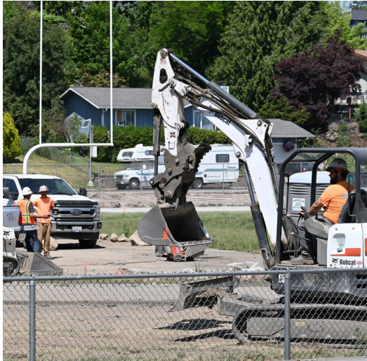
Cheney High School Stadium Renovation progress on June 18.
