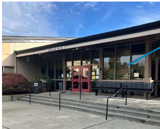
BLDG 100 - MAIN ENTRY
