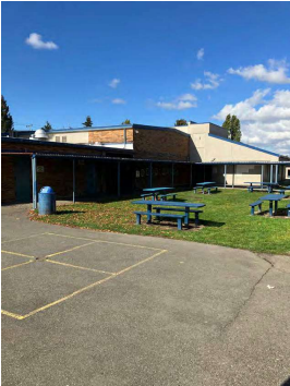
BLDG B - COURTYARD
