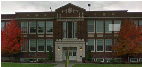
CONSTRUCTION PERIOD 1900-1940'S
