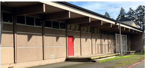
CONSTRUCTION PERIOD 1940'S-1970'S
