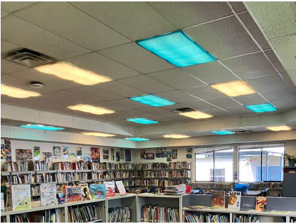
BLDG C - LIBRARY
