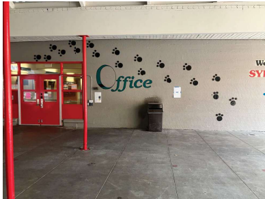
BLDG 100 - MAIN ENTRY
