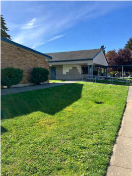
BLDG C - MAIN ENTRY
