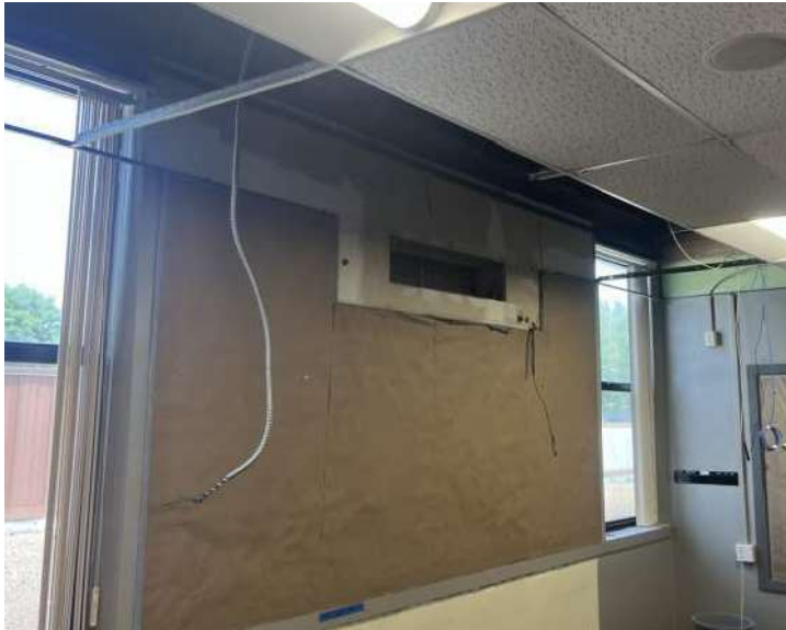
Ridgeview - Existing HVAC Unit Removal
