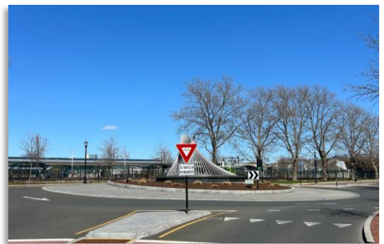
Roundabout at Bank St and Columbus Blvd
