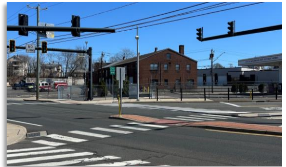
Refuge area on E Main St at CTfastrak
