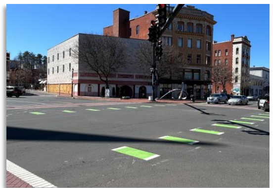
Pavement markings at Arch St and Main St
