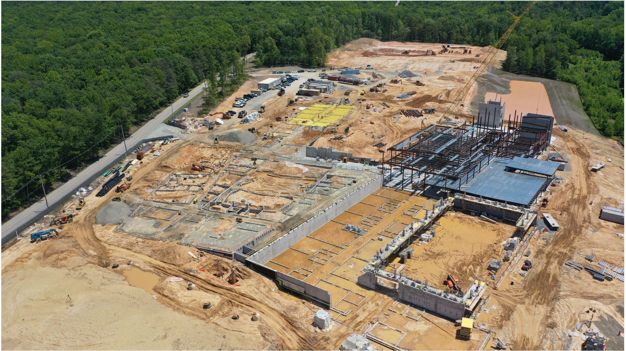
NORTH EAST MIDDLE / HIGH SCHOOL – REPLACEMENT
