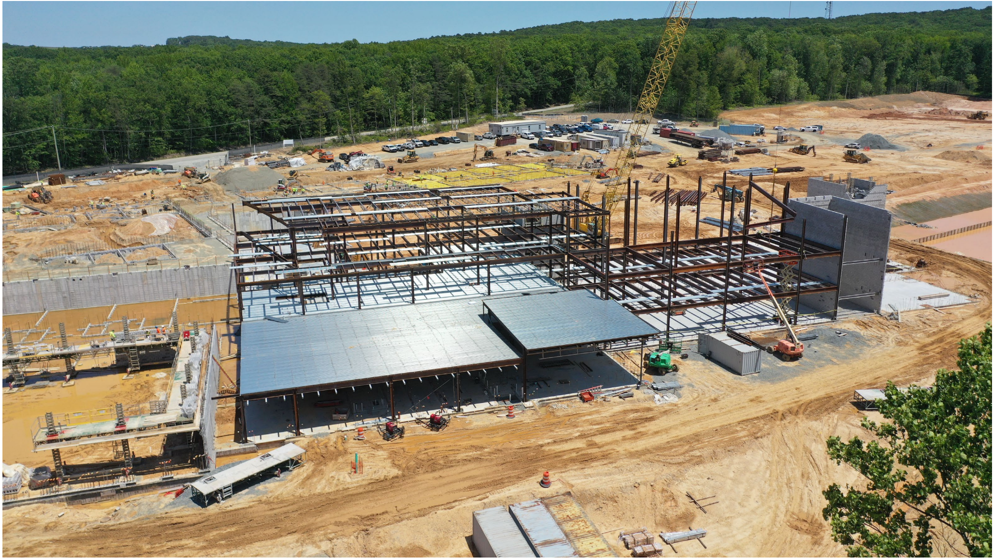
NORTH EAST MIDDLE / HIGH SCHOOL – REPLACEMENT
