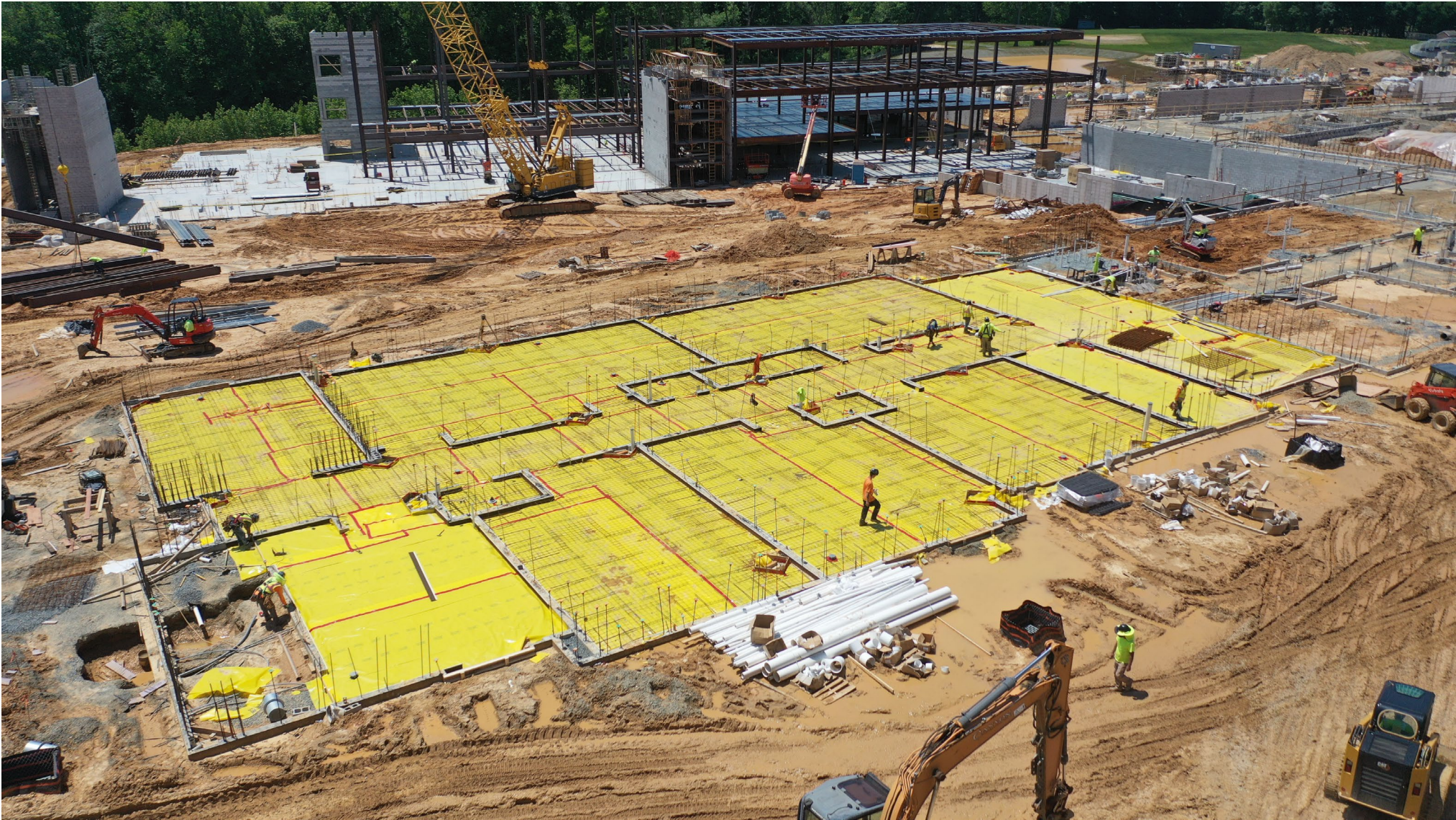
NORTH EAST MIDDLE / HIGH SCHOOL – REPLACEMENT
