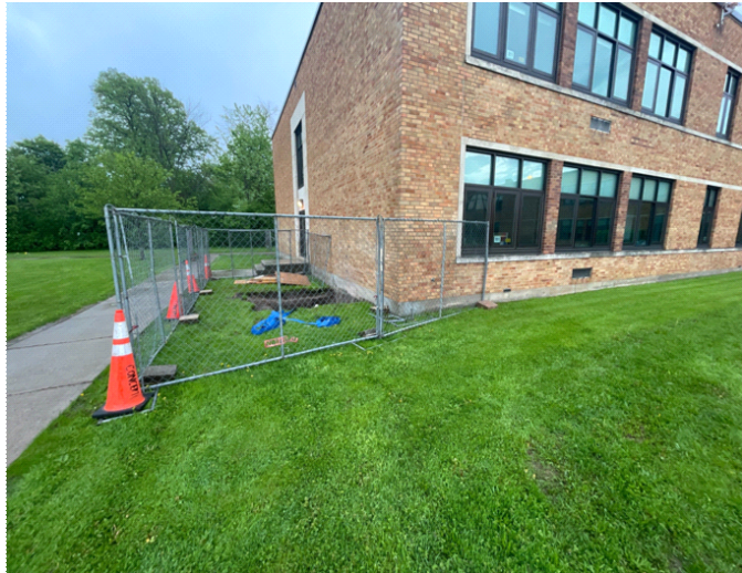
MS - Asbestos abatement access points & negative air exhausts
