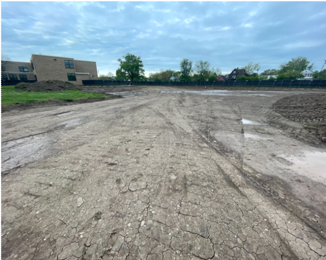
New UPK Addition @ WBS - Site preparation / temporary fencing
