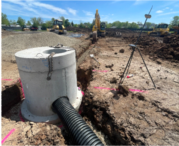
New UPK Addition @ WBS - Storm drainage and structures installed.
