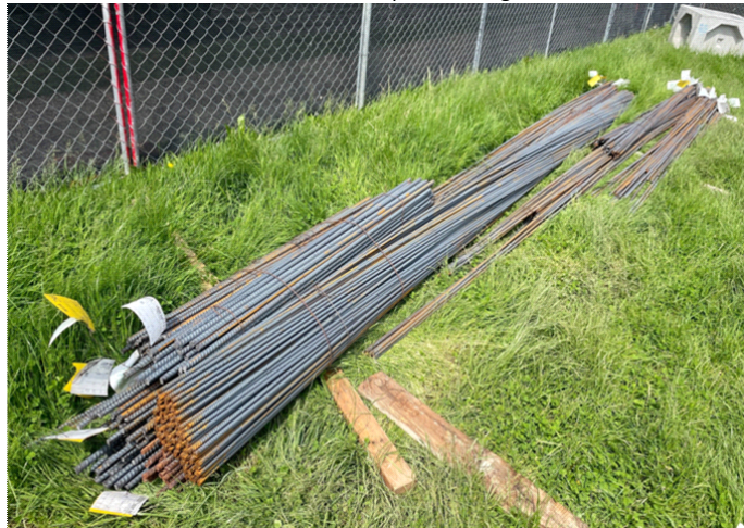
New UPK Addition @ WBS - Rebar staged for new bldg. foundations
