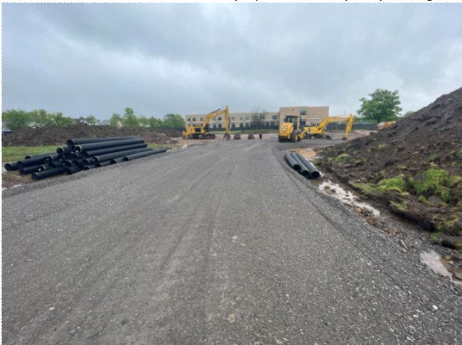
New UPK Addition @ WBS - Stone subbase for construction access / new drop off loop
