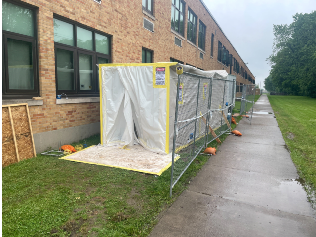
MS - Asbestos abatement decontamination areas at the crawlspace.
