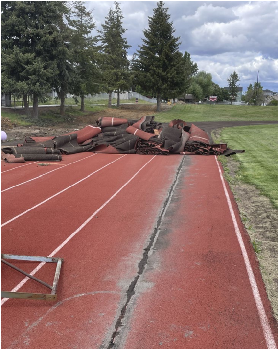
Track Surfacing Demolition
