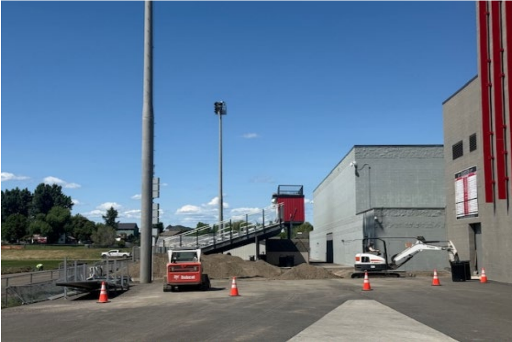
Demolition of Asphalt for Bleacher Pad
