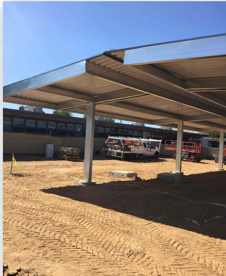
Construction of lunch shelter
