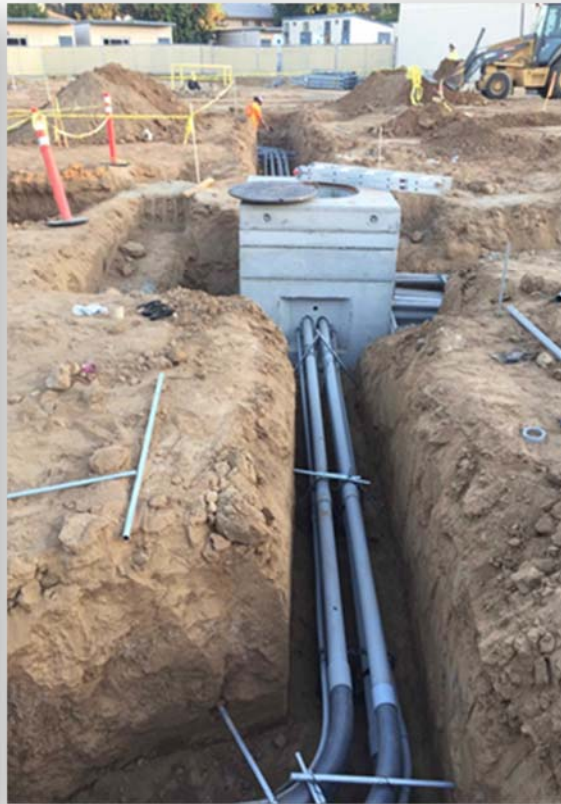
Gas line, electric conduits and storm drain encasing
