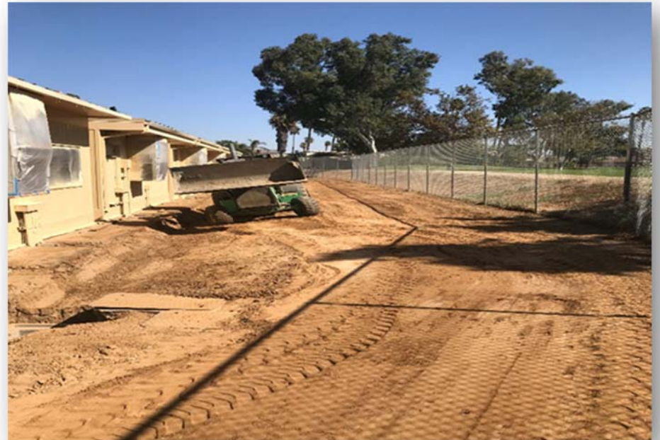
Final grading at the portables
