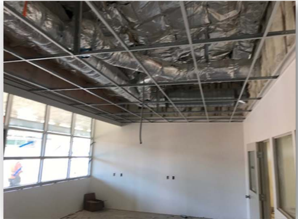
Building D1 roof installation and ceiling grid
