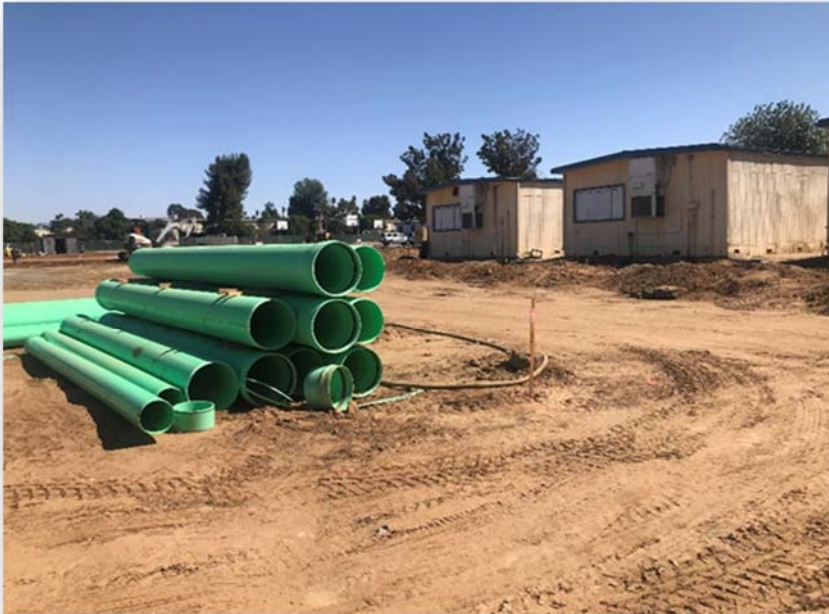
Storm drain installation
