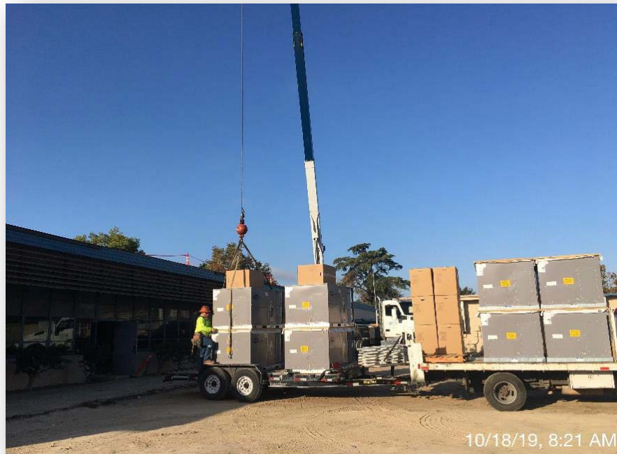
New AC units for Buildings D & E were delivered to the site
