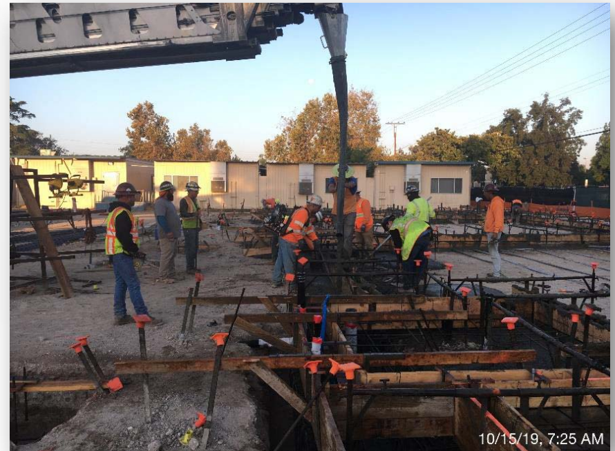
Concrete pour at the new Kindergarten Building
