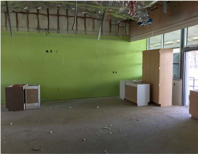
Casework and paint in Building C1
