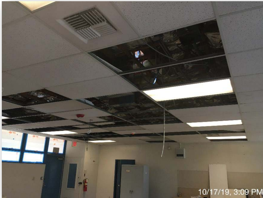
Installation of the new lights
