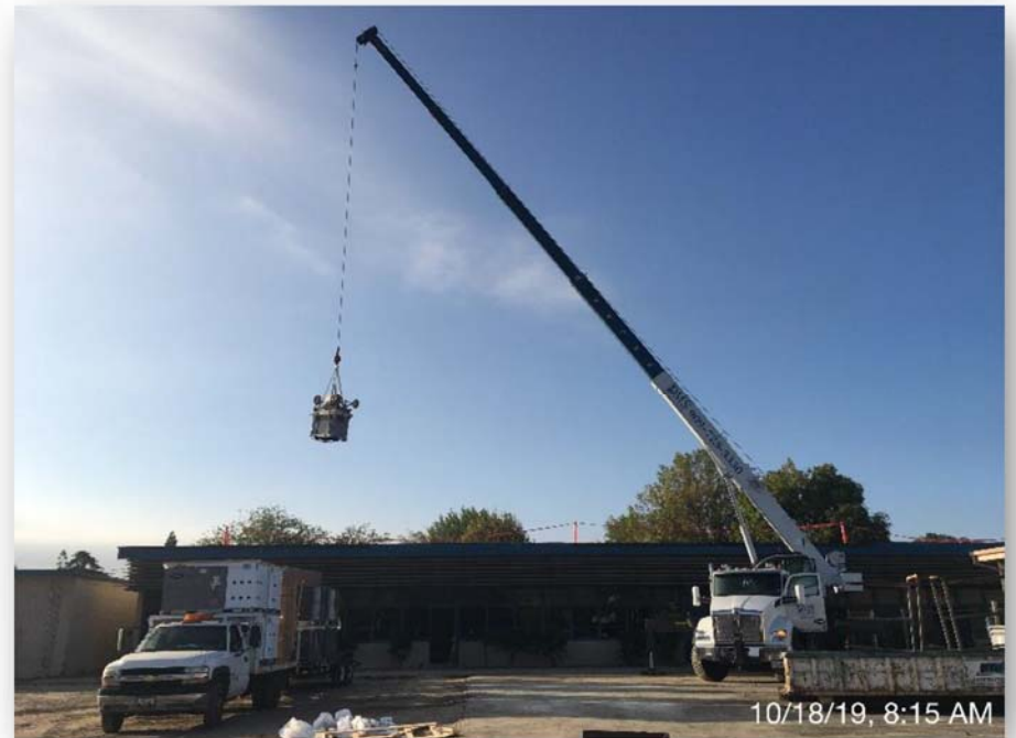
New AC unit craned to the roof of Building D
