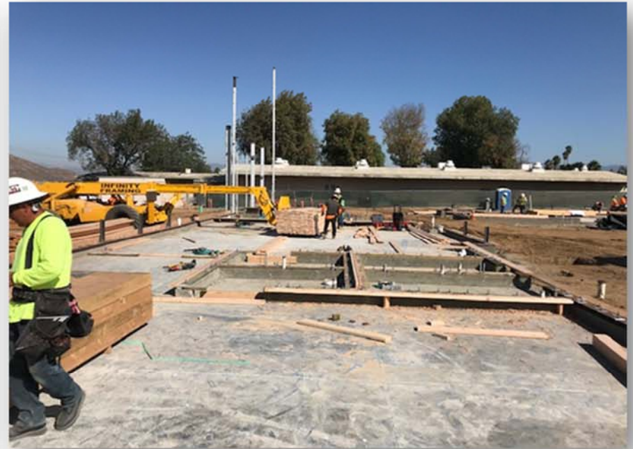
Slab work and framing in Building F2
