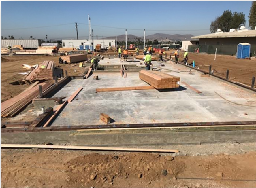
Slab work and framing in Building F2
