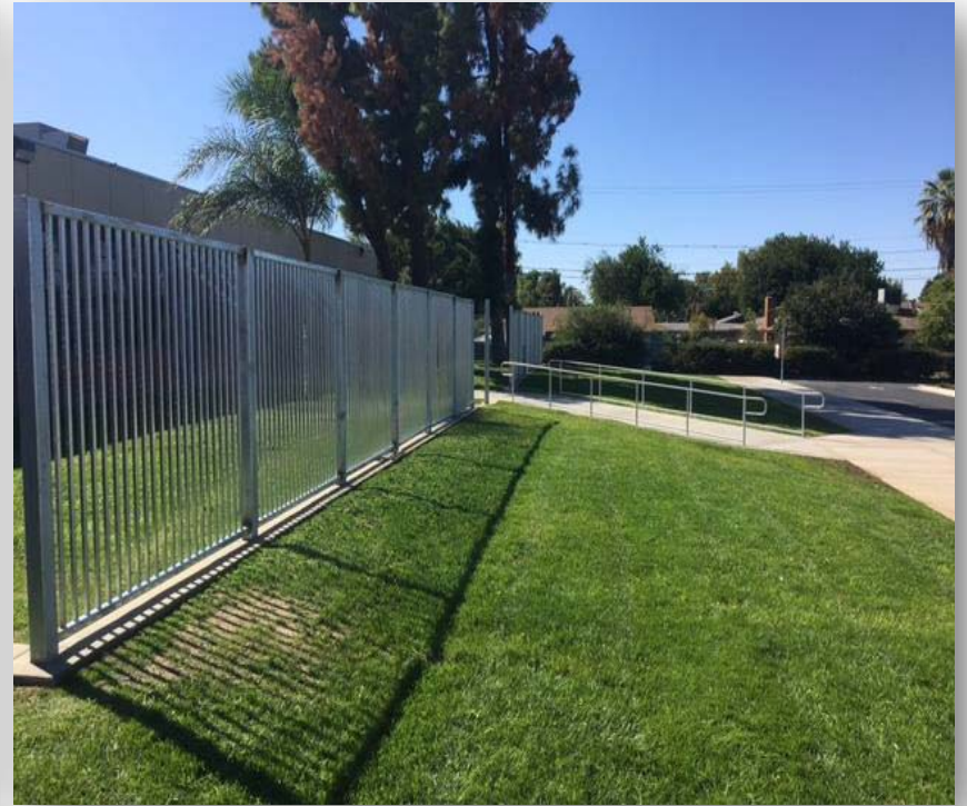
Front fence and handrails
