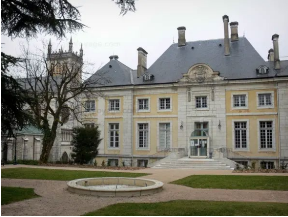
The exterior of the school in Belley France
