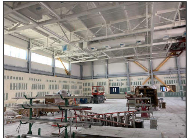
New Gym Building – Interior drywall finish and paint
