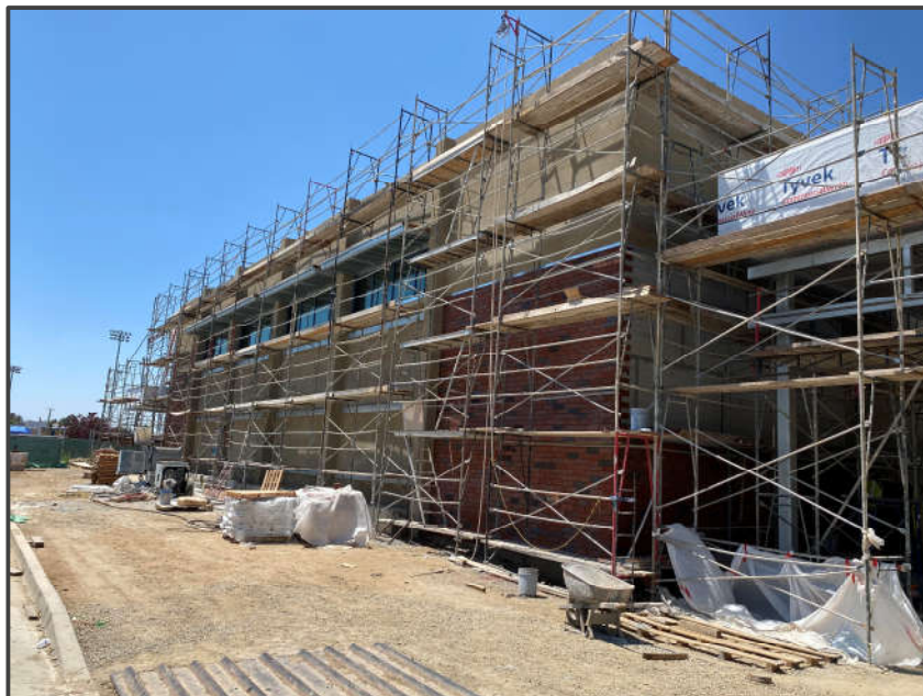
New Gym Building – Window glazing and brick veneer
