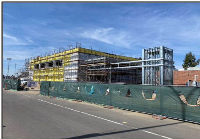
New Gym Building – Ongoing roofing, metal lath and scaffolding
