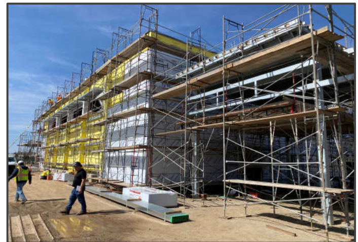
New Gym Building – Ongoing roofing, metal lath and scaffolding
