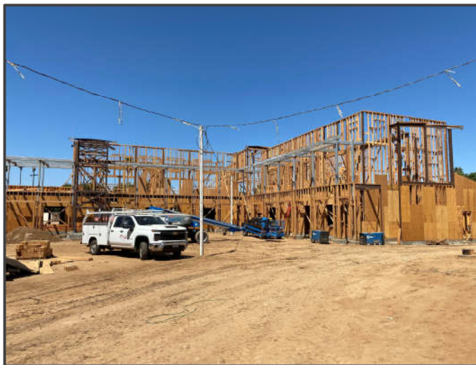
East 2-Story Classroom Bldg. F – Wall framing, plywood sheathing & MEP rough-in
