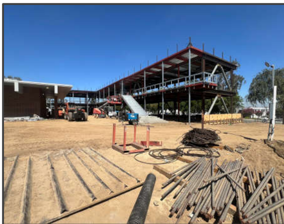
New 2-Story Science Classroom - Ongoing steel decking, railing & stair installation work
