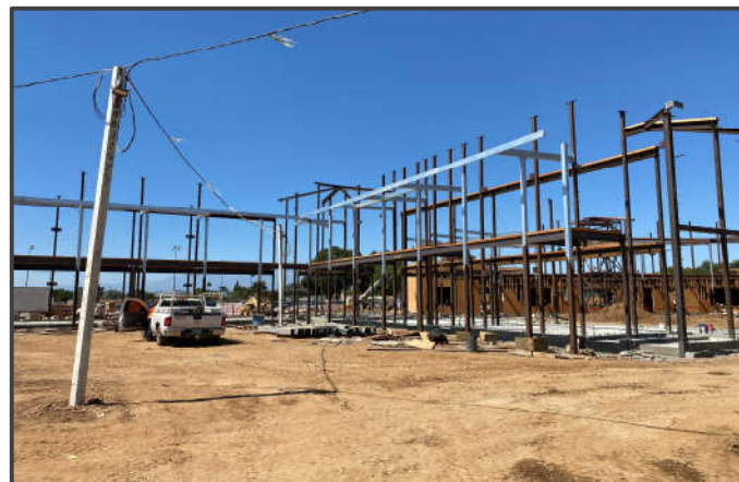
West 2-Story Classroom Bldg. D – Structural steel welding, slab on grade clean up for base plating
