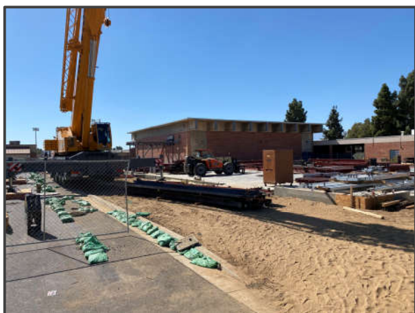
New Gym – Crane set up for the structural steel erection
