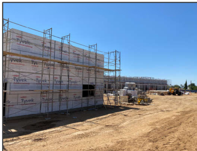
Kindergarten Bldg. C – MPE rough-in, Tyvek, roofing, and metal lath
