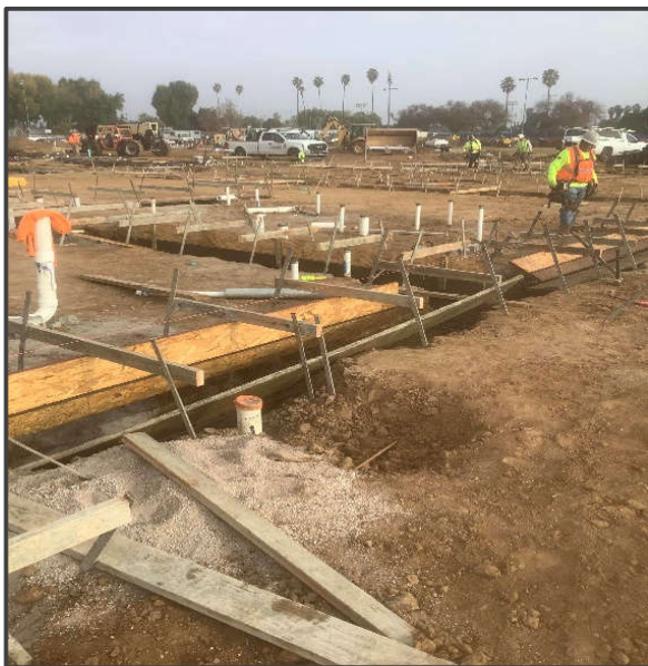
Bldg. B – Foundation Form Setting
