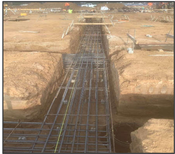
Bldg. B – Foundation Steel Reinforcement Placement
