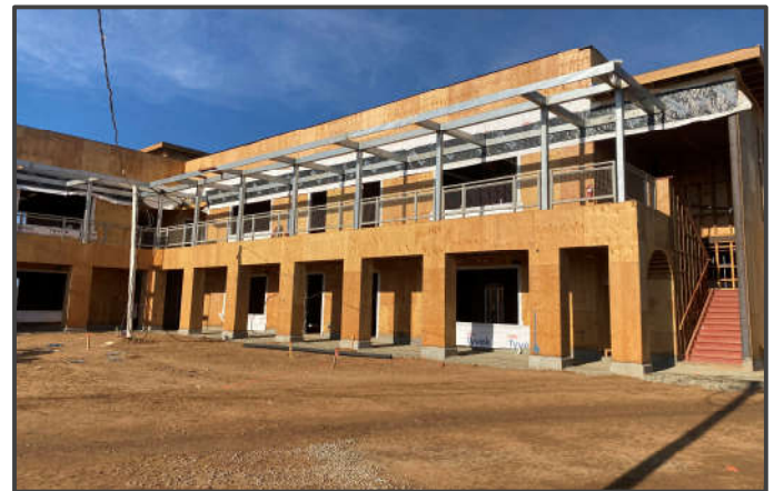
West 2-Story Classroom Building D – Roofing, plywood sheathing, MEP rough-in & door-window frame work
