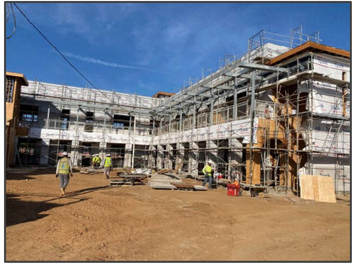
East 2-Story Classroom Building F – Prep work for stucco & drywall work
