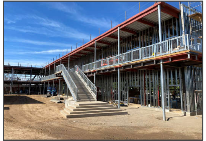
New Science Classroom Building – Metal stud framing & MEP rough-in work
