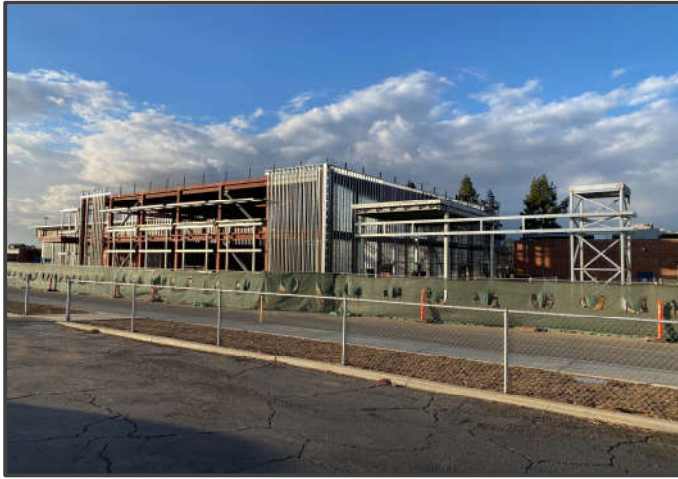
New Gym Building – Metal stud wall & signage steel framing work
