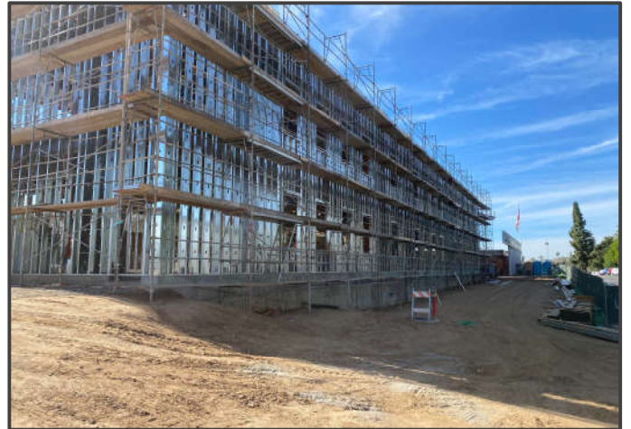
New Science Classroom Building – Metal stud framing work
