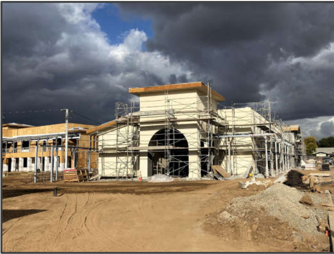
Admin Building A – Stucco color coat work
