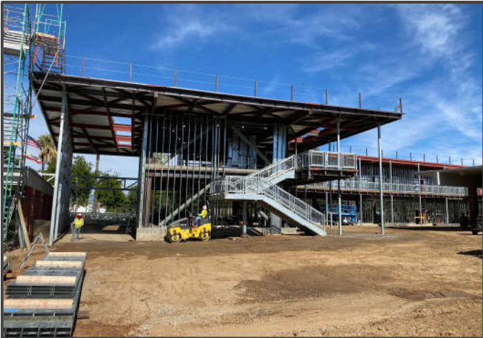
New Science Classroom Building – Metal stud framing & MEP rough-in work
