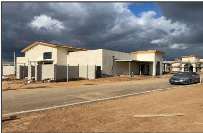
MPR Building B – Concrete block enclosure work
