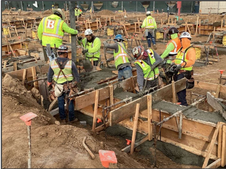
Pouring Concrete into Footing
