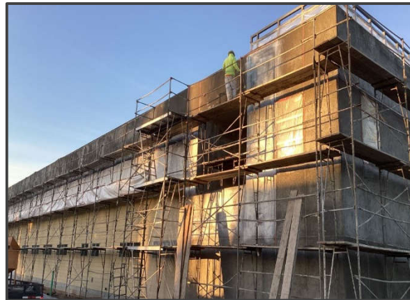
Plaster & Siding on 2-Story Bldg.
