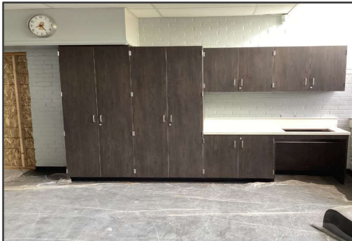
Casework Installation
