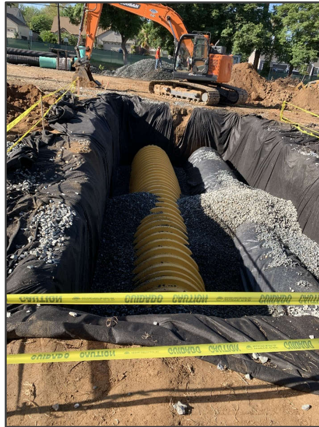
Underground Storm Retention
