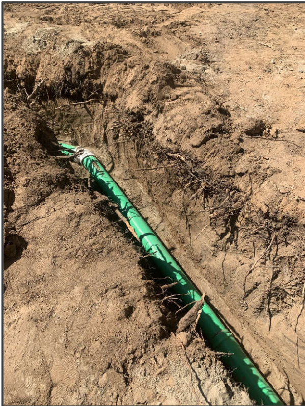
Underground Storm Water Pipe
