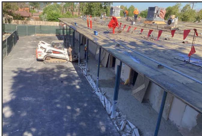
Demolished Roof and Path of Travel Concrete
