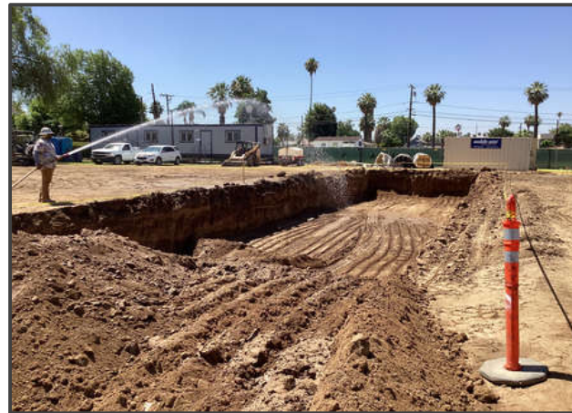
Over-Excavation for New Modular 2-Story
