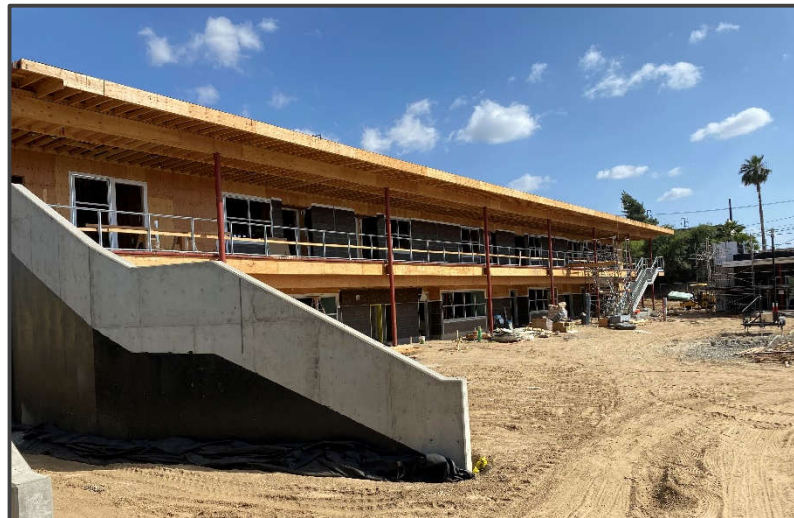
Single Story Building K2 Pre-Work for Stucco Installation
