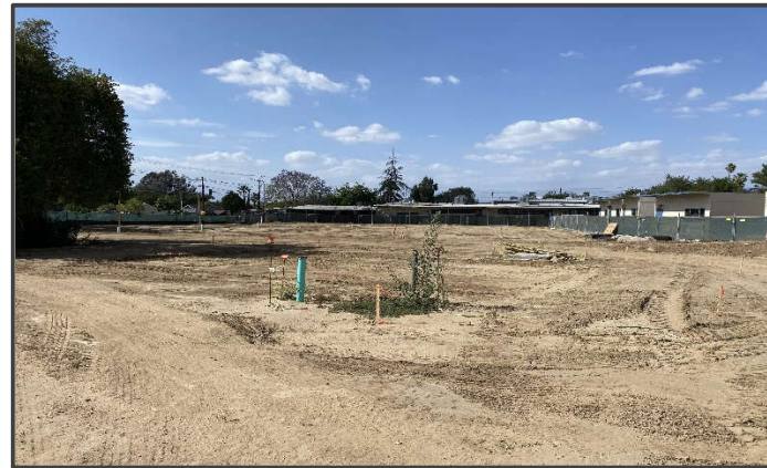
Grading for Portable Classroom Relocation
