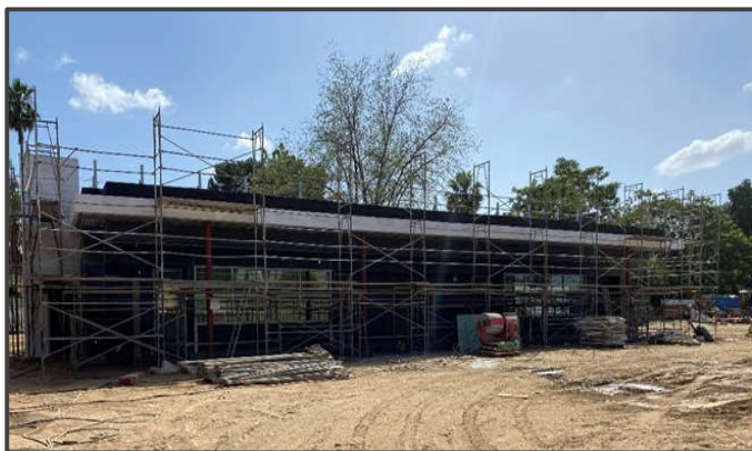
Single Story K2 Pre-Work for Stucco Installation
