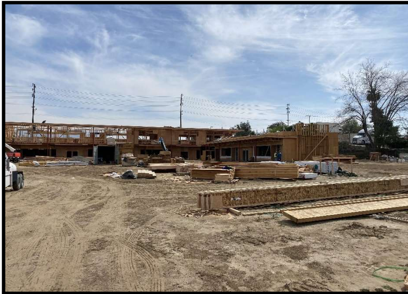
Building K1 & K2 Steel & Wood Framing
