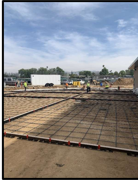
Prepping for Hardscape/Concrete
