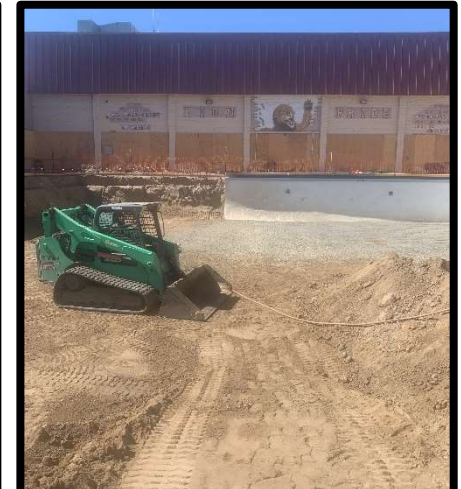
Pool Backfill
