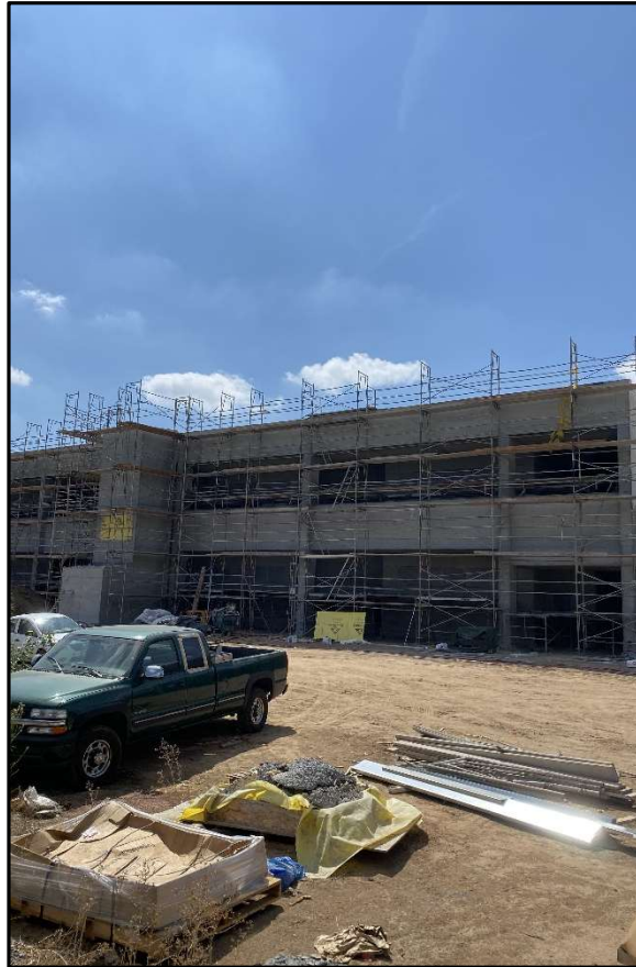
Building J Stucco Scratch Coat Installation
