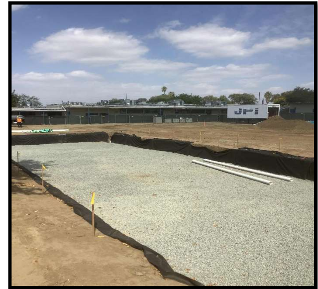
New Drain Retention Basin
