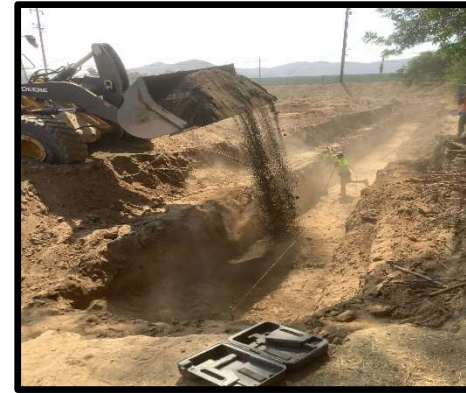
Storm Drain Easement Trenching
