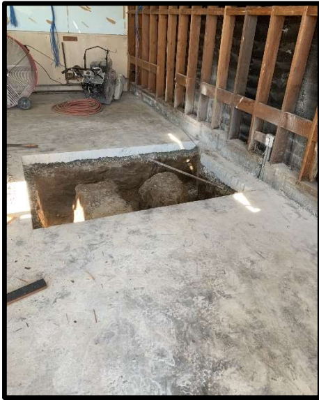
Restroom Slab Work
