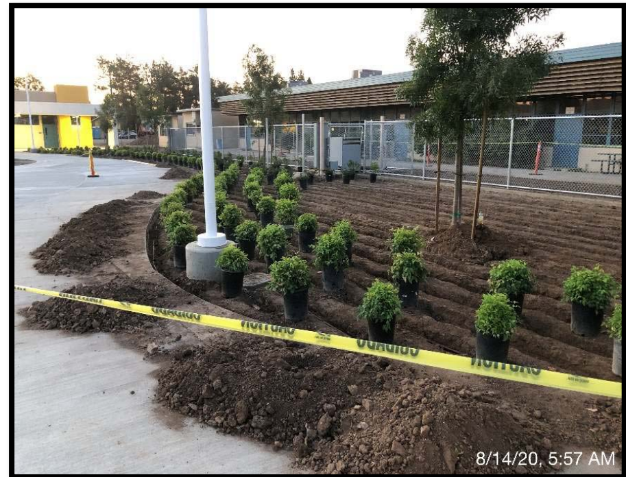
irrigation lines and planting
