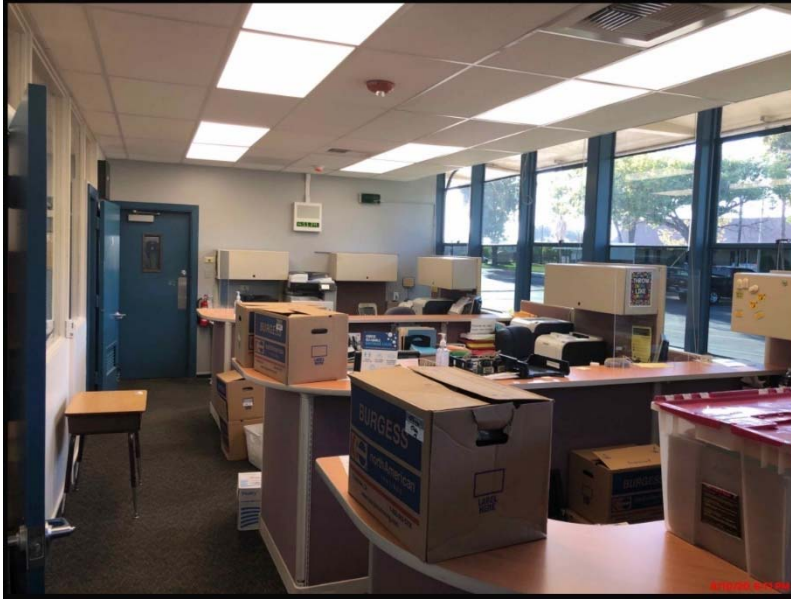
Administration area work complete including new light fixtures, fire alarm, ceiling grid and tiles, HVAC, and roofing
