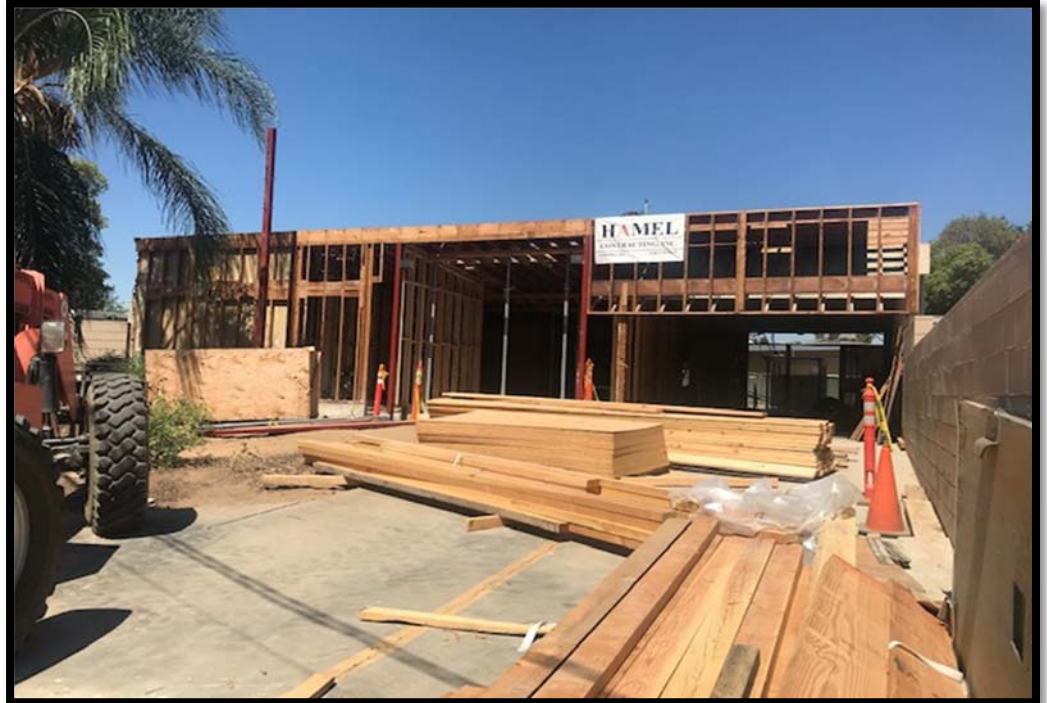
Existing administration building with façade demolished
