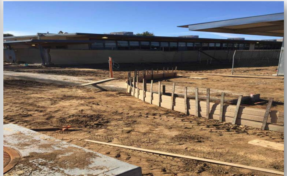
Building G Footings
