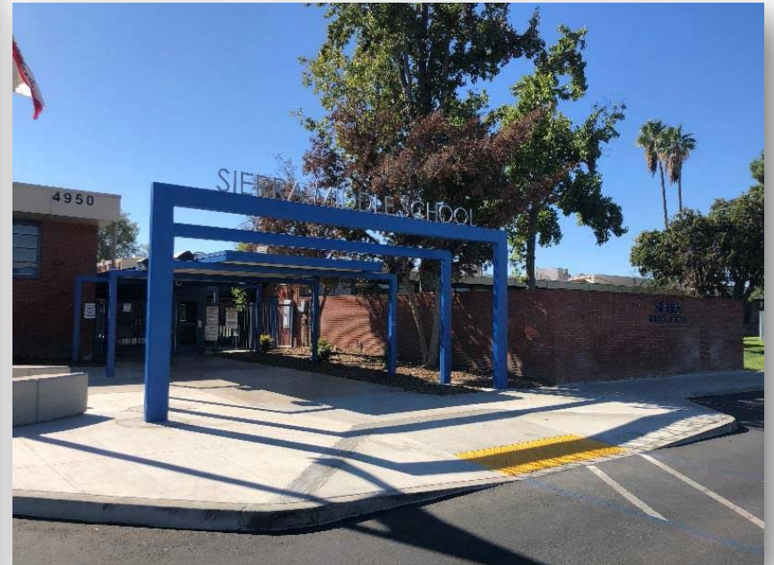
Front fence and handrails
