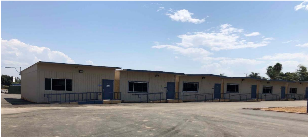
Completed interim housing portables
