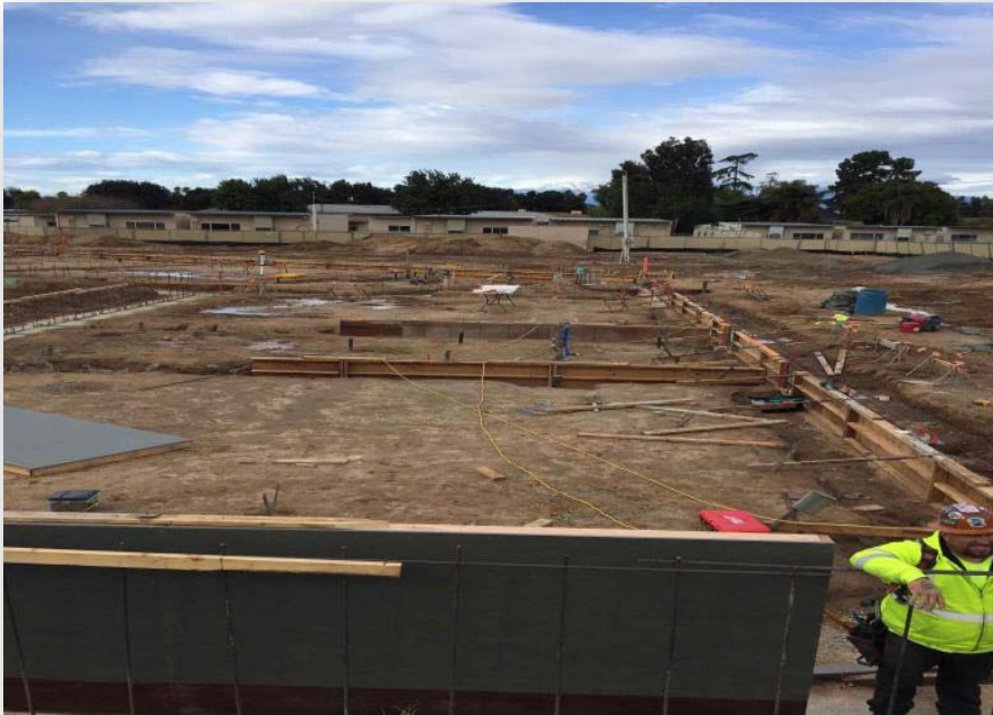
Set Forms & Clean Footings
