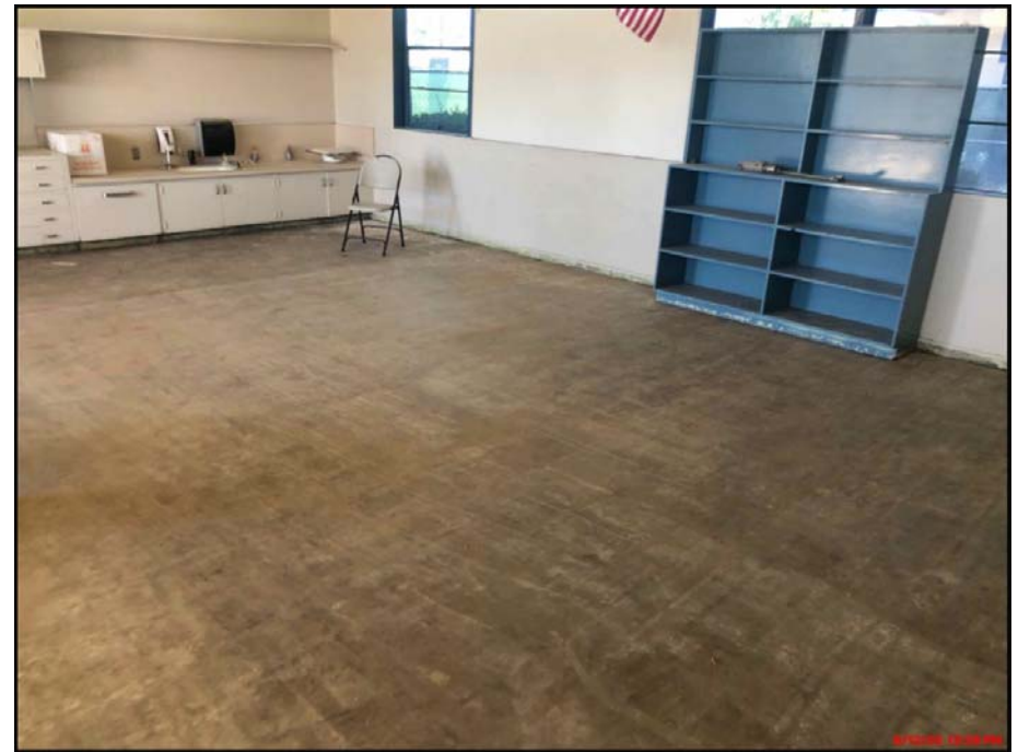
Phase 2 demolition is complete which includes the renovation of two classrooms buildings
