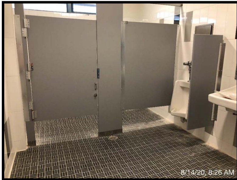
Ceramic tile installation at the restrooms in the Admin Building
