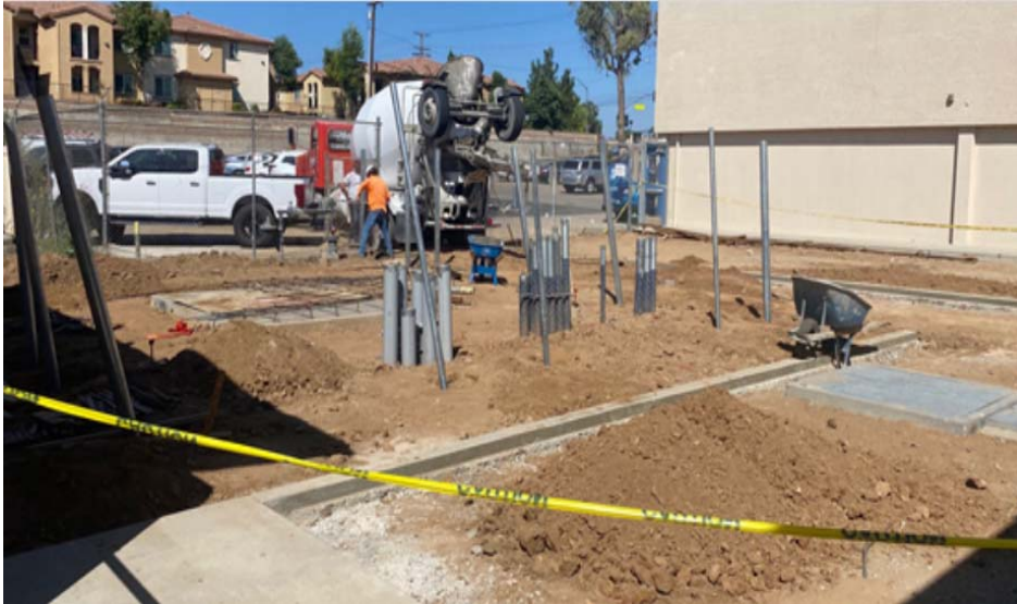
Electrical utility sweeps installed for new electrical utility yard
