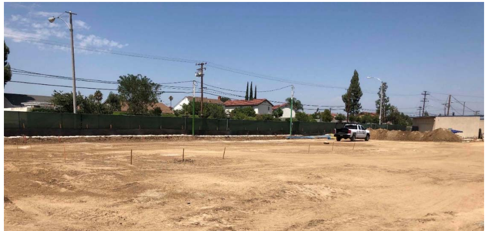
Ongoing grading operation for the new building
