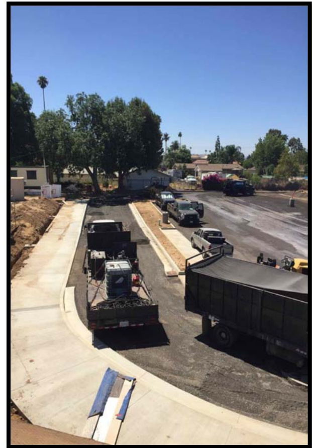
Prep for asphalt
