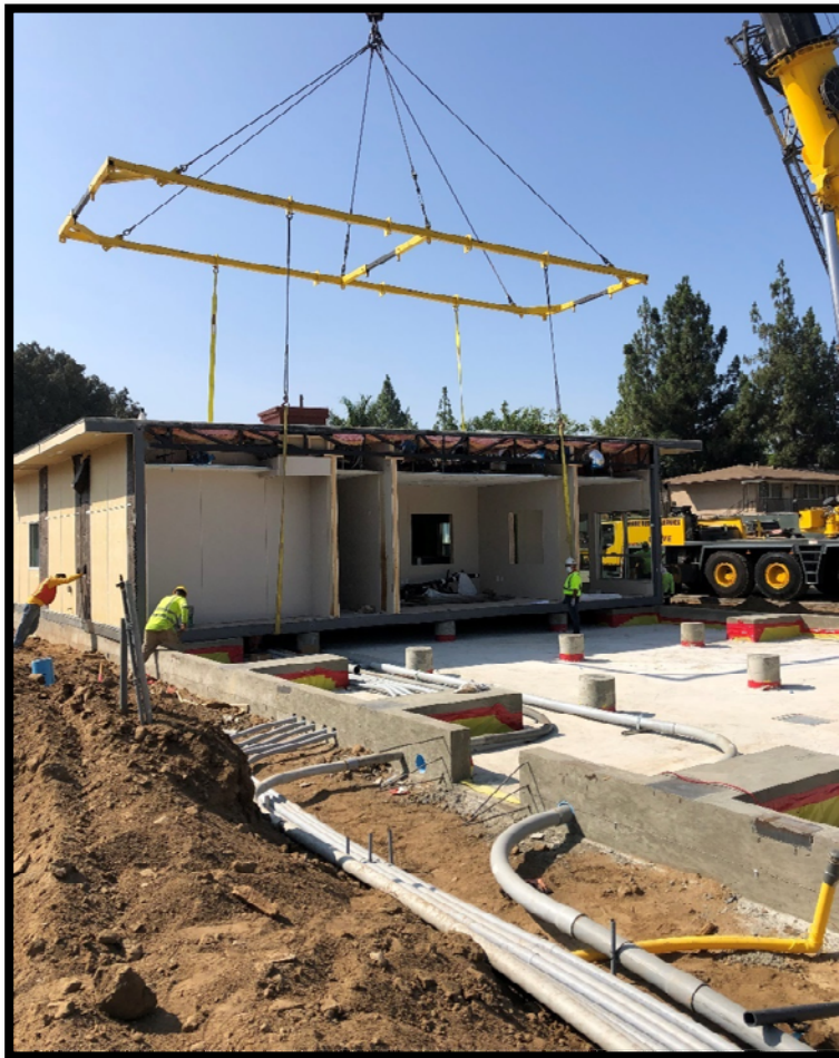
Building C crane operations
