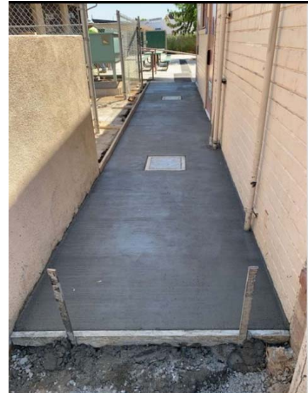
Gas line installed and poured back
