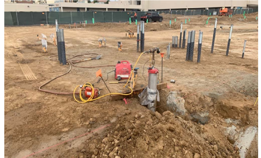
Grading complete for new Kindergarten building, underground utilities for installed and backfilled at the new building
