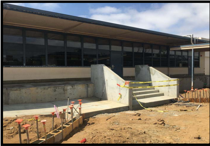
New Ramp & Stairs
