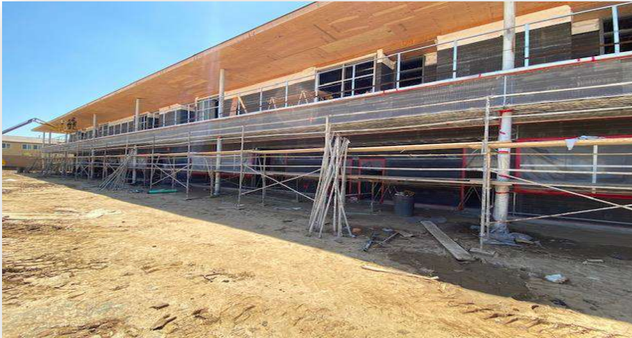
First floor of the East Elevation is ready for the scratch coat of the plaster system
