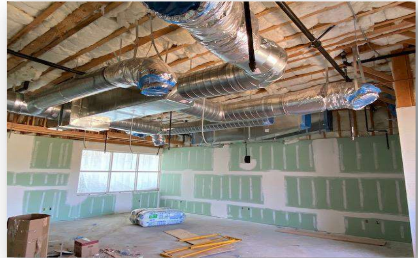
Mechanical duct work is being installed
