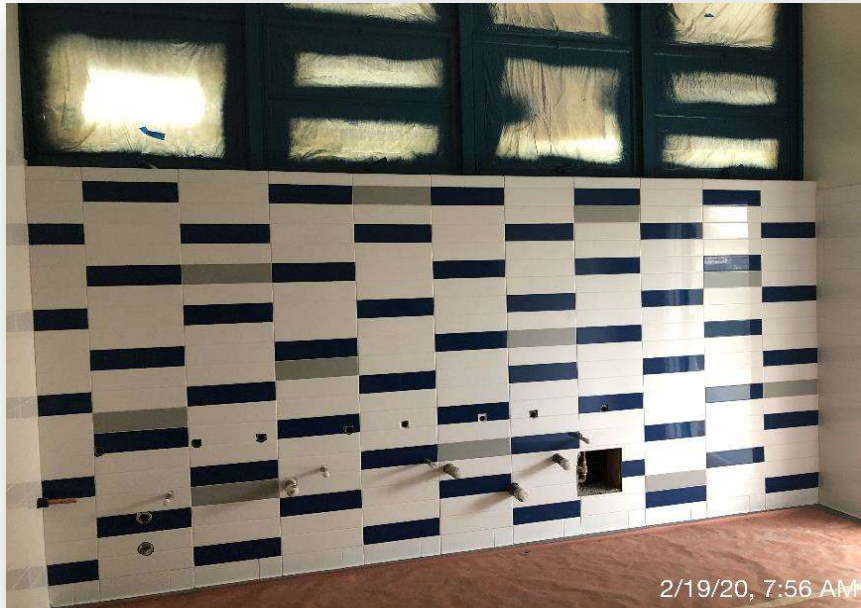
Ceramic tile installation
