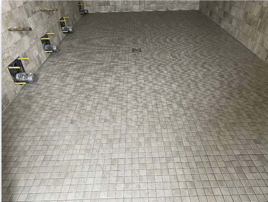
Tile installation in new restrooms at Building D
