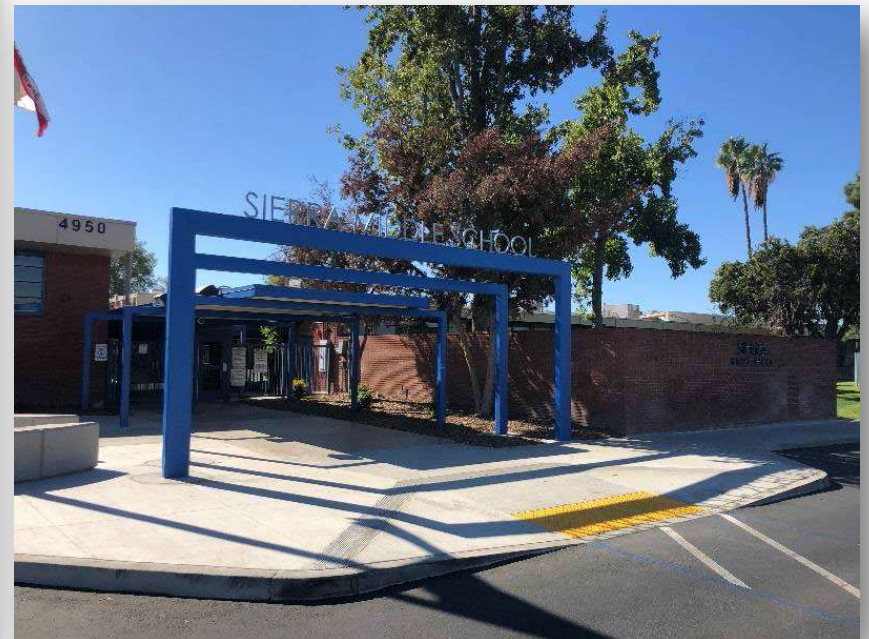
Front fence and handrails
