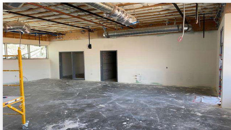
First floor classrooms are ready for paint & t-bar
