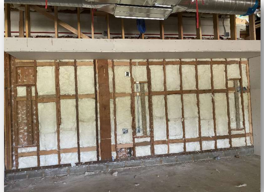
Wall & roof installation in kinder classrooms
