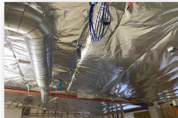
Wall and roof installation in kinder
