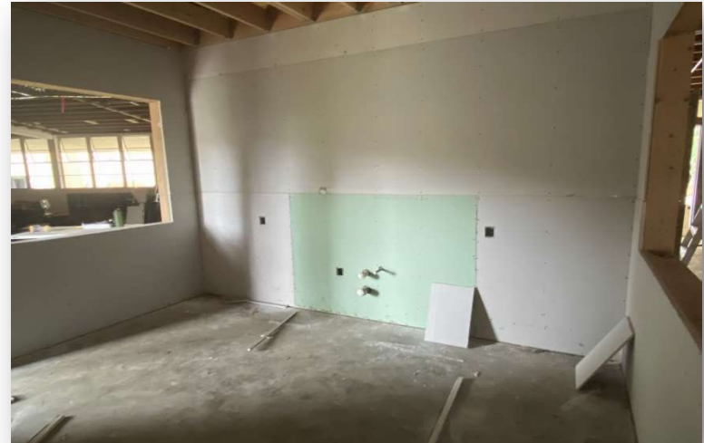
Drywall at kinder classrooms, workrooms & restrooms
