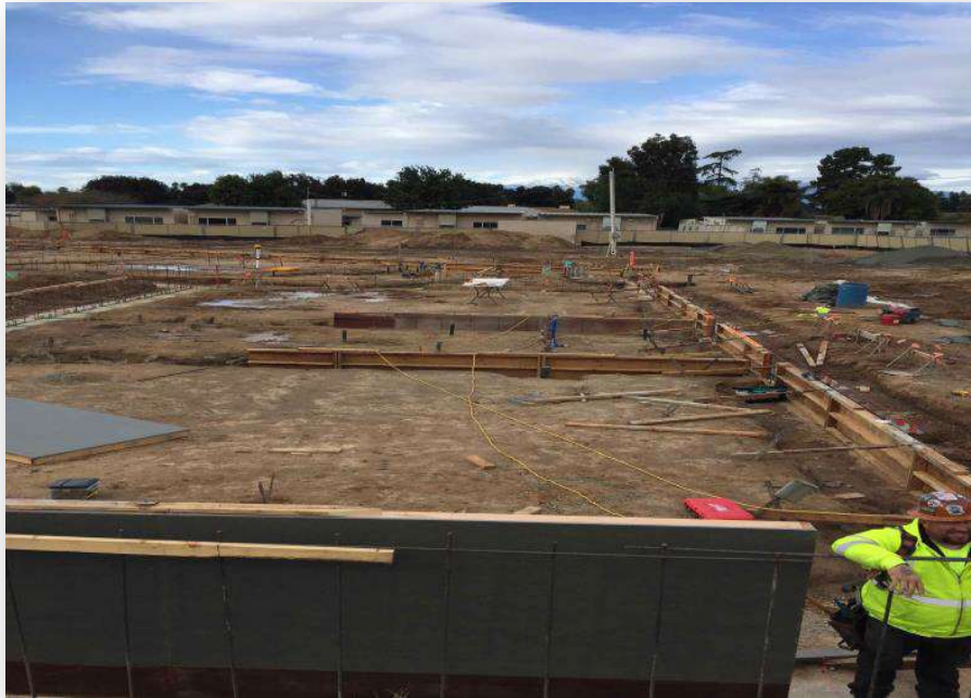
Set Forms & Clean Footings
