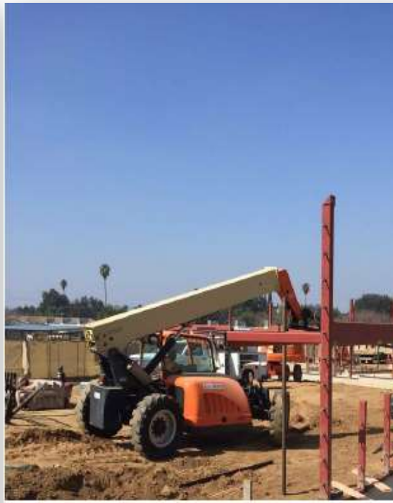
Steel work & framing
