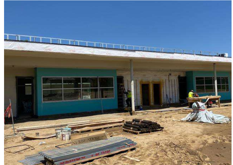
Exterior window systems are being installed
