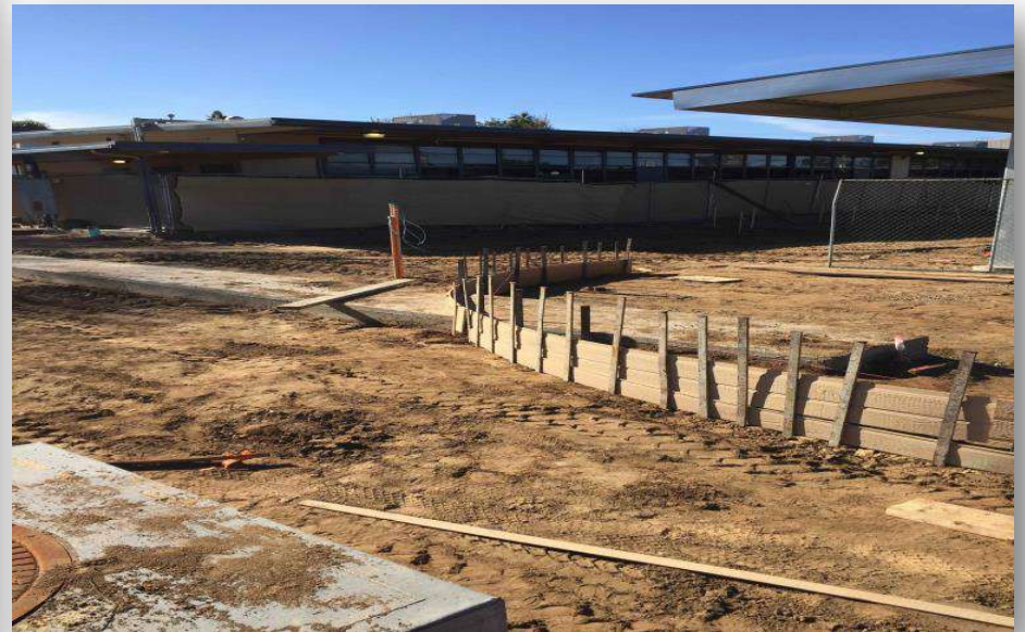
Building G Footings
