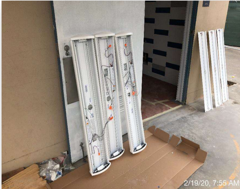
New light fixture installation
