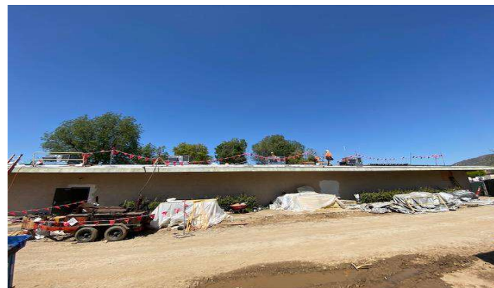
Cap sheet on the roofing system
