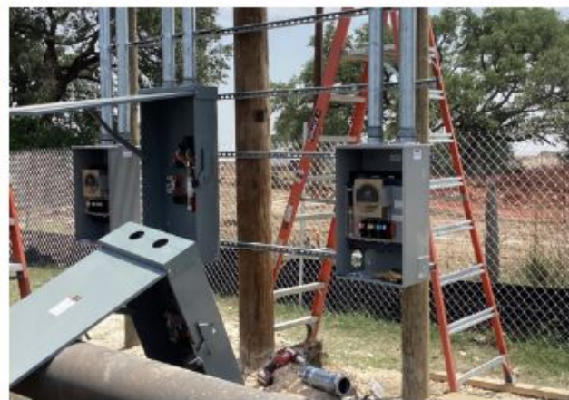
Installing Temporary Power Panel
