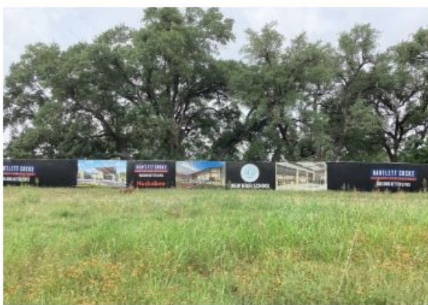
Installed Windscreen @ Jobsite Perimeters
