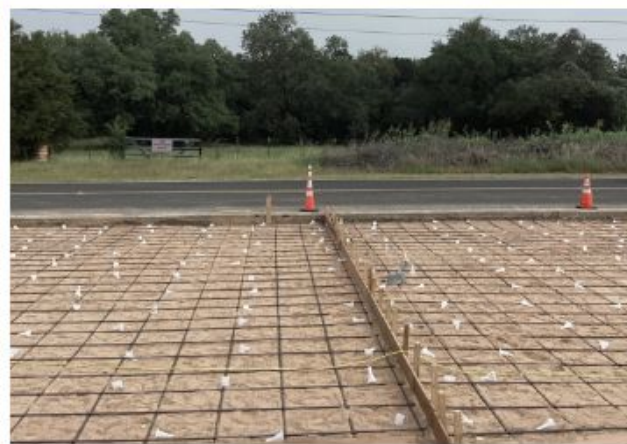
Placing Rebar for Approach Entrance #01
