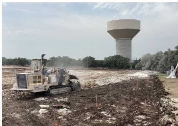
Excavating Building & Site
