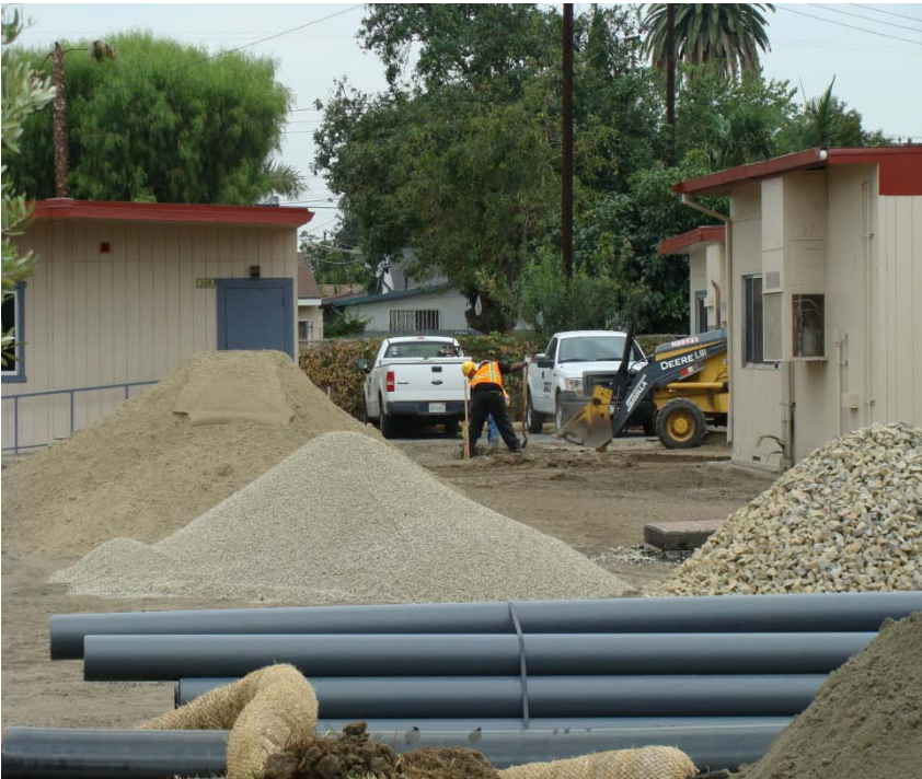
Drain line pipes
