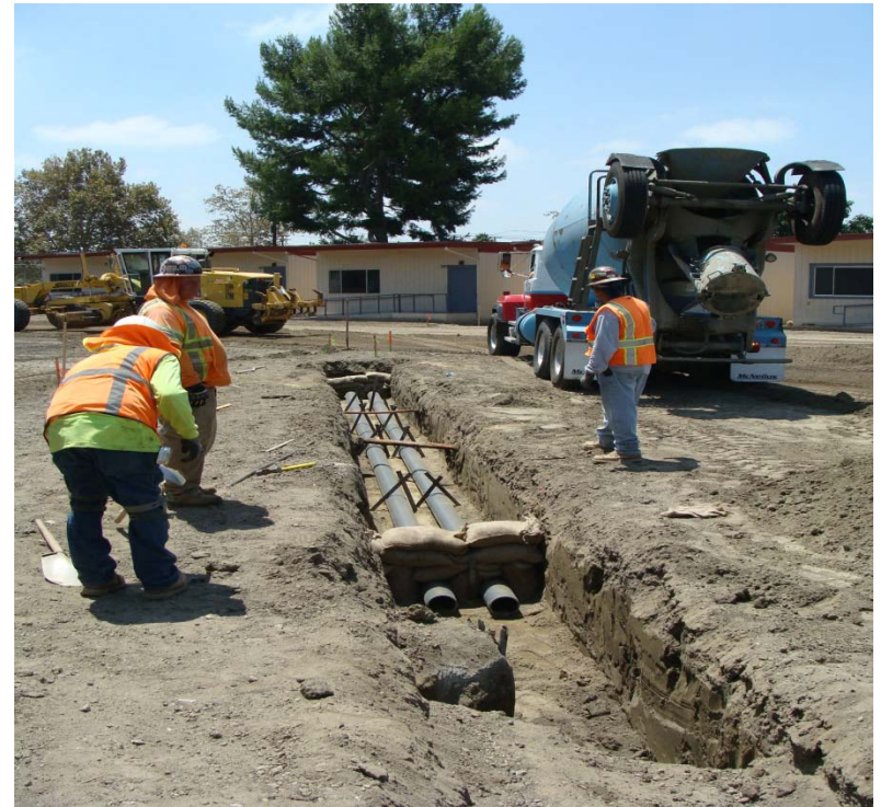
Installation drainage system
